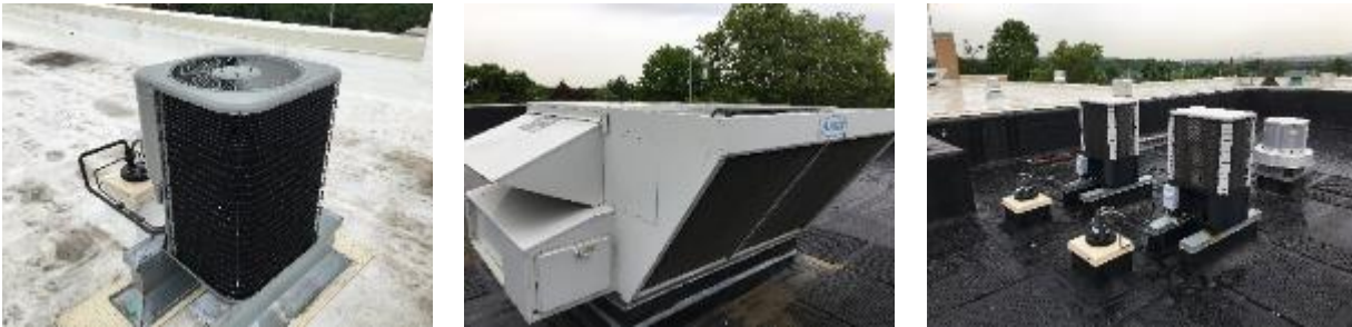
Image 4: Air Conditioning Systems
