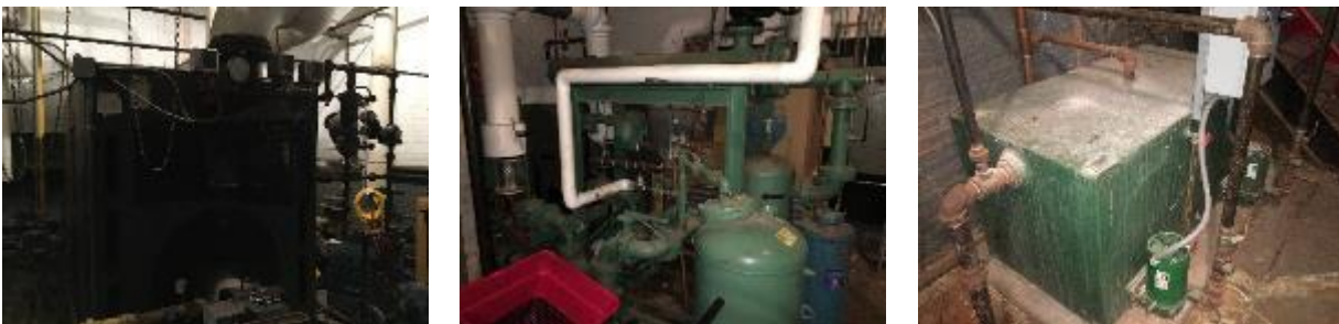
Image 3: Steam Heating System
