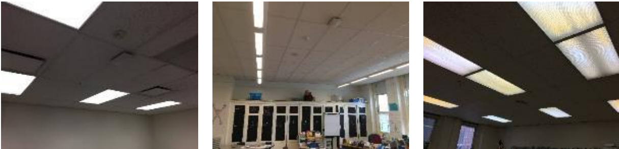
Image 2: Interior Lighting Systems
