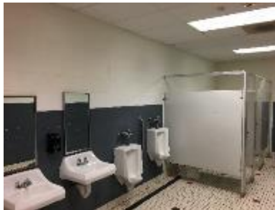
Image 9: Water Using Systems
