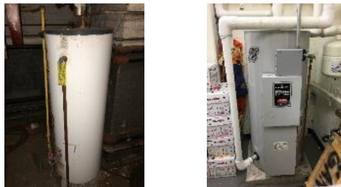
Image 5: Domestic Water Heating Systems
