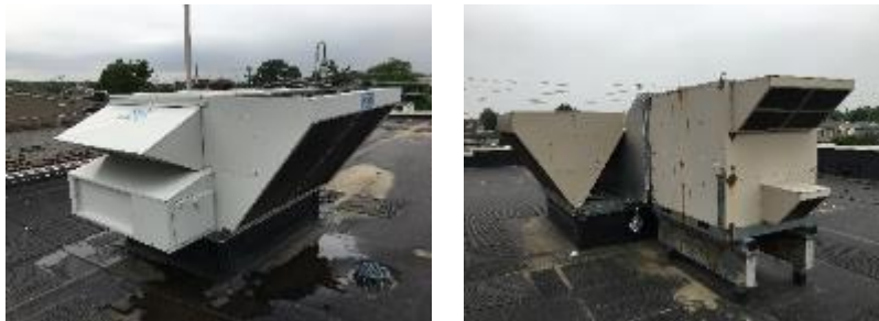
Figure 9 – Rooftop HVAC Equipment
