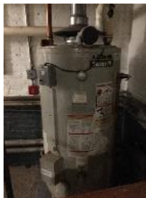
Figure 10 – Domestic Hot Water System Equipment
