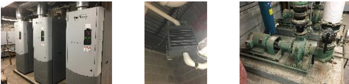
Figure 10 – Heating Hot Water Equipment
