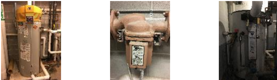
Figure 13 – Domestic Hot Water Equipment
