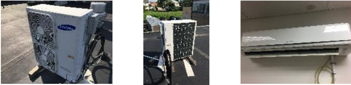
Figure 12 – Air Conditioning Equipment
