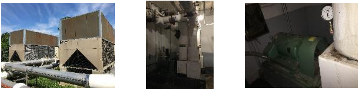
Figure 9 – Chilled Water Equipment
