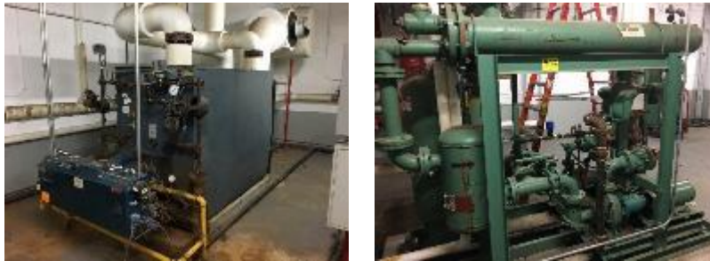
Image 3: Hot Water Heating System
