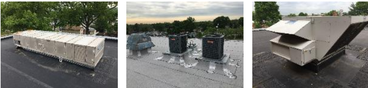
Image 4: Air Conditioning Systems
