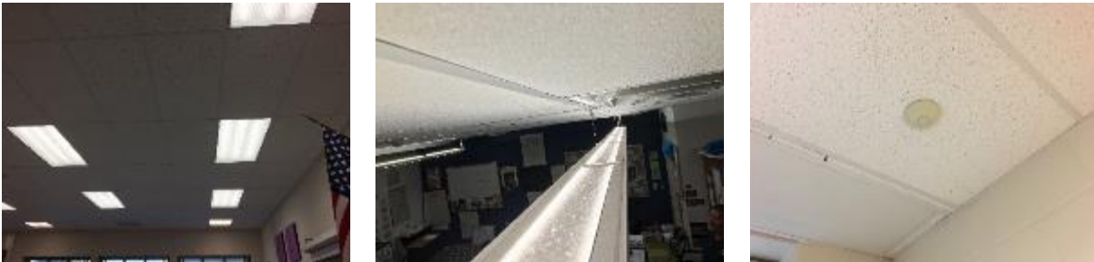
Image 2: Interior Lighting Systems
