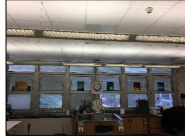
Lighting control in most spaces is provided by wall switches. There are occupancy sensors installed in the teachers' lounge, two administration office restrooms and four student restrooms. Stairwells, elevator lobbies and main lobby areas do not contain any occupancy sensors and operate continuously throughout the day until the evening maintenance staff leaves the building after their shift.
