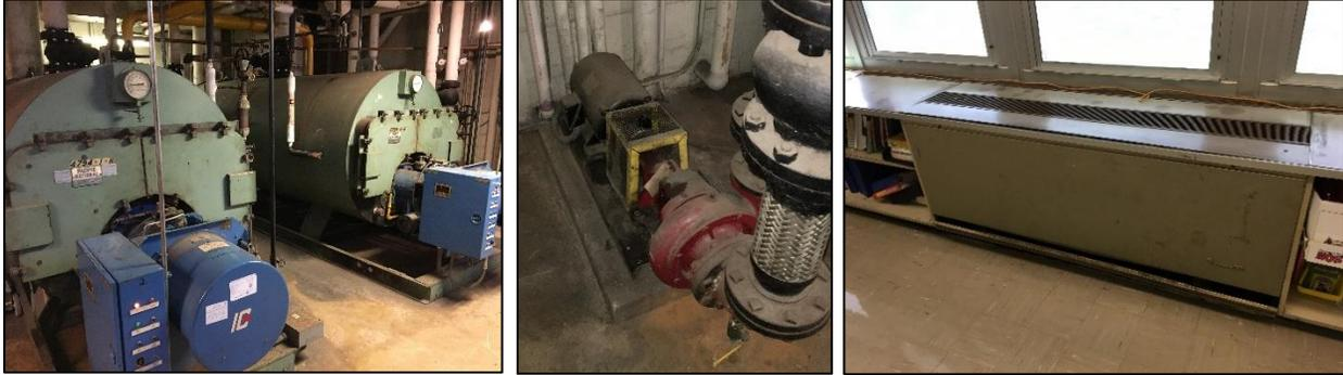
The boilers operate in a lead/lag configuration. Both boilers may be required during cold weather. The lead boiler is rotated weekly.
