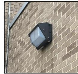
The building's exterior lighting consists primarily of efficient LED fixtures that are controlled by photocells, though there are a few fixtures with high pressure sodium lamps, compact fluorescent lamps, and incandescent lamps that are controlled by schedule timers.
