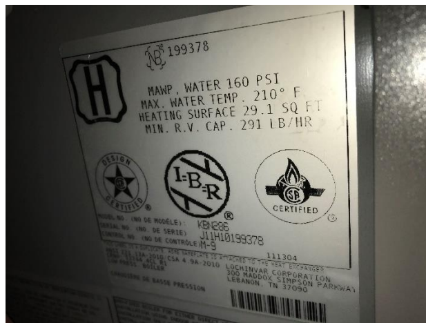
Image 3 Boiler nameplate
