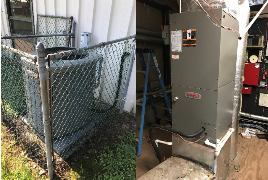
Image 4 Building Cooling and Heating System
