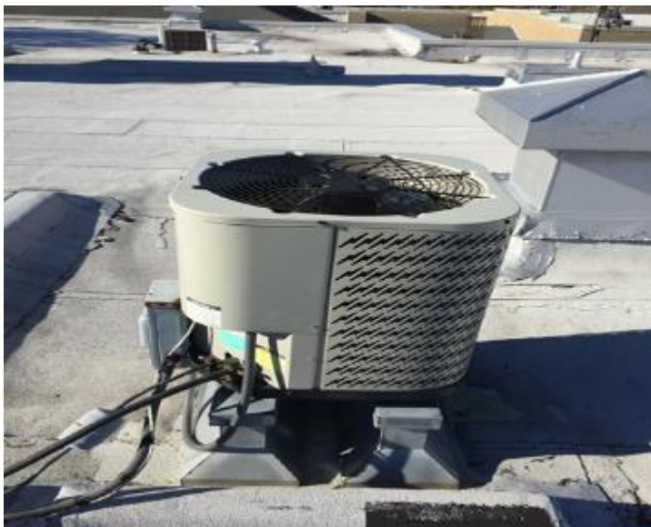
Image 3: Air Conditioning System
