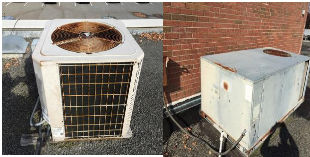
Image 2: Air Conditioning Equipment
