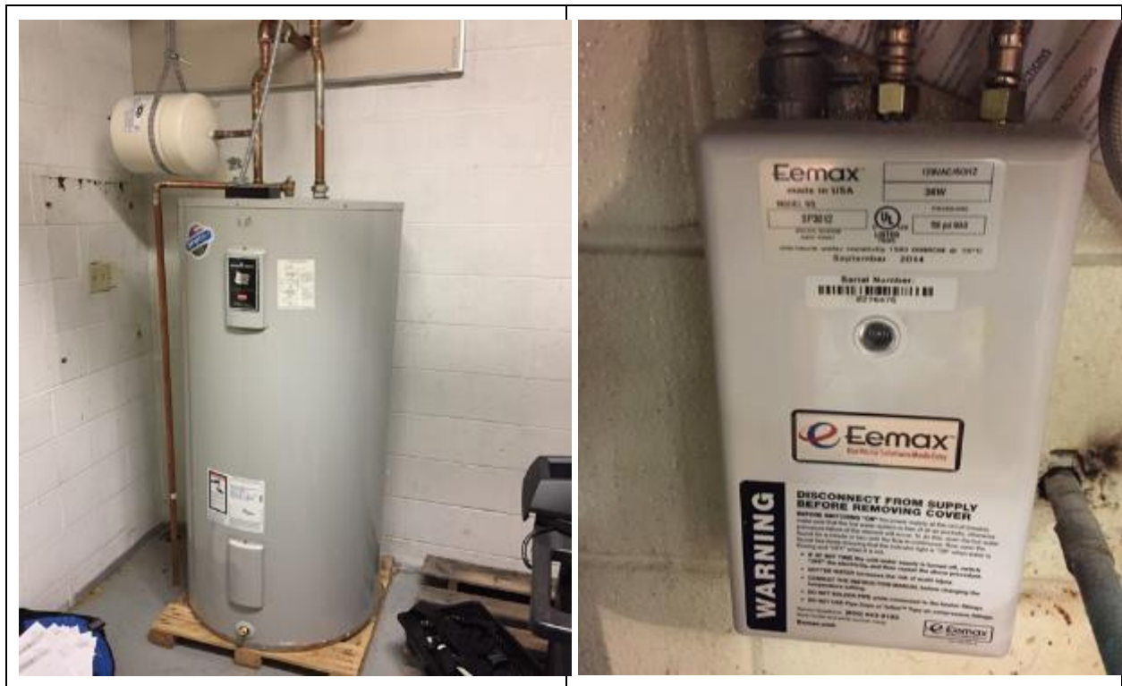
Image 3: Domestic Hot Water
