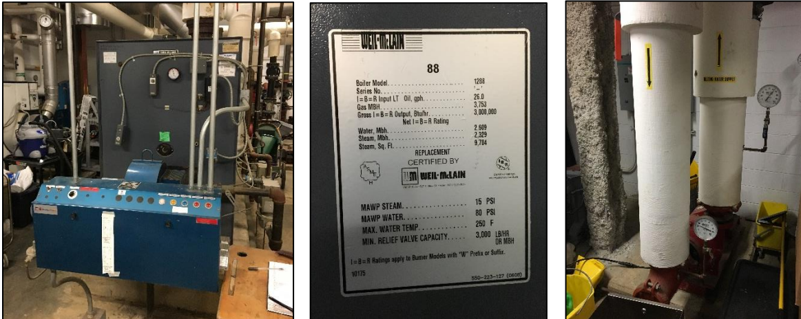
Image 3: Hot Water Heating
