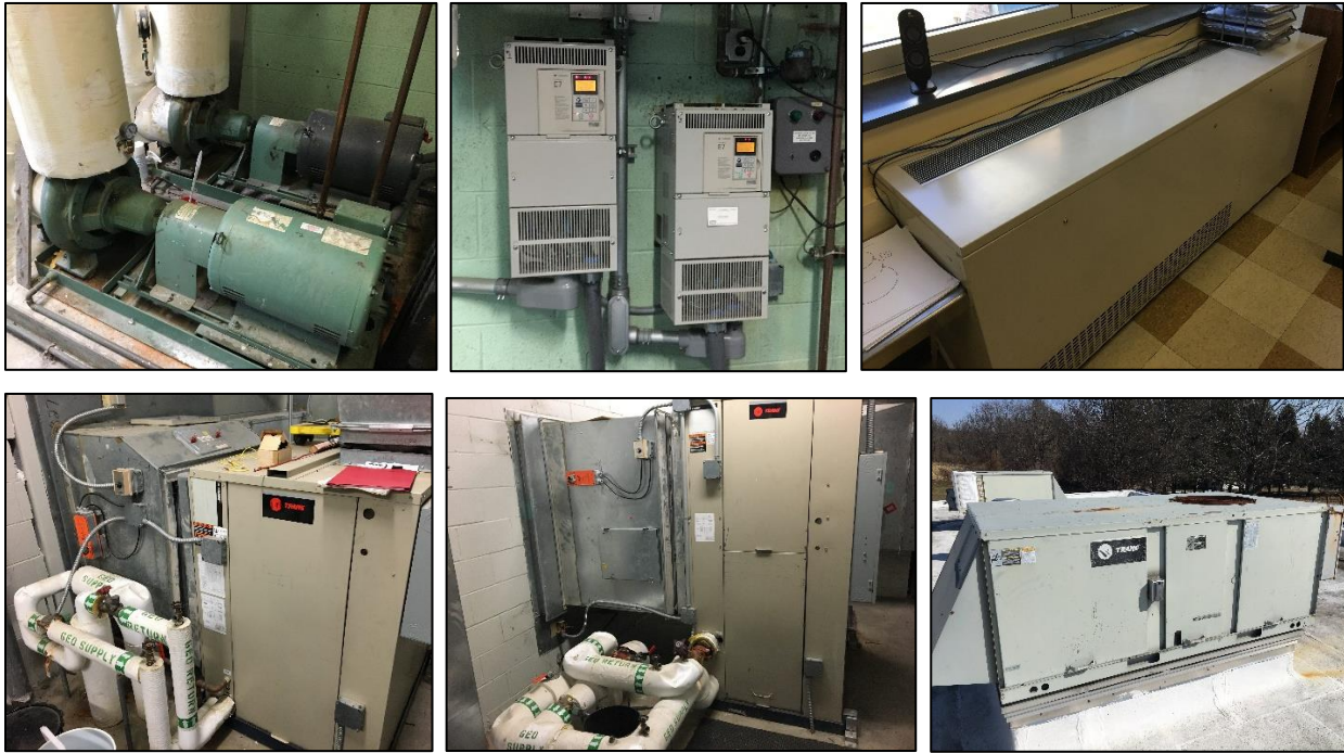
Image 4: Ground Source Geothermal Water Loop System
