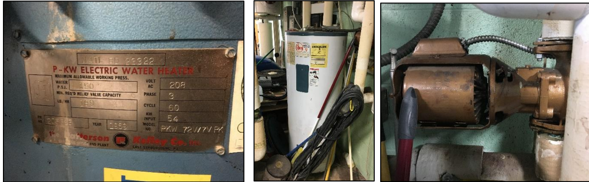
Image 7: DHW Heating System
