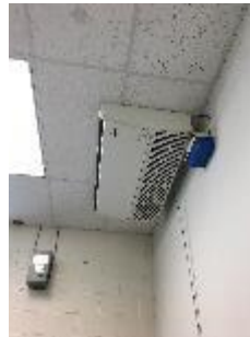
Figure 13 – Air Conditioning Equipment
