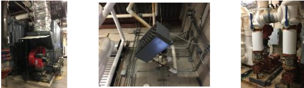
Figure 11 – Hot Water Heating Equipment
