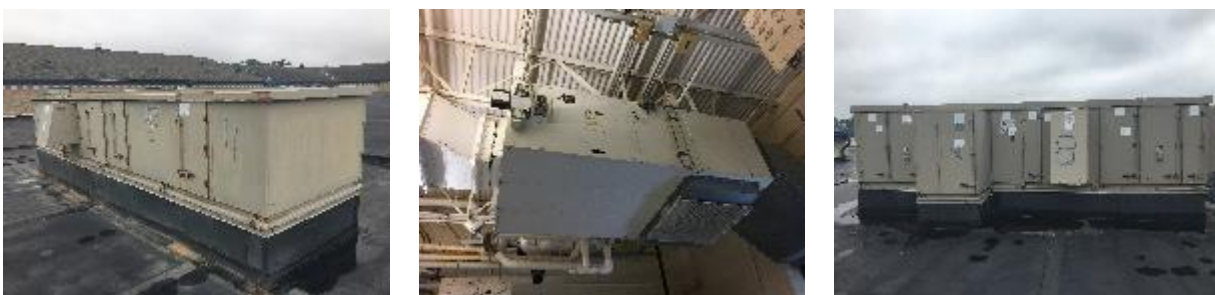
Figure 12 – Air Conditioning Equipment
