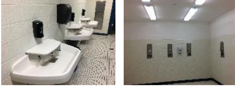
Figure 19 – Water Using Equipment
