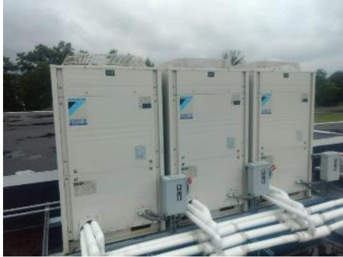
Fig 5a – Kitchen Office (Mitsubishi City Multi) Fig 5b – A Wing: Split Systems (Daikin VRV)
