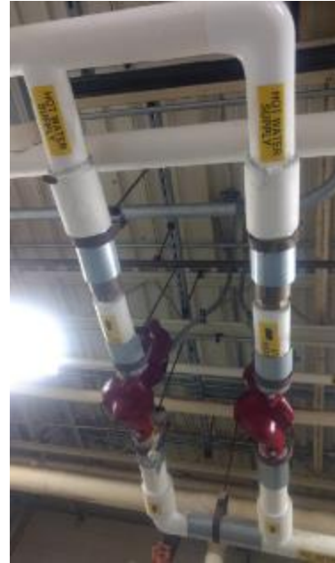
Fig 4b –Hot Water Pumps
