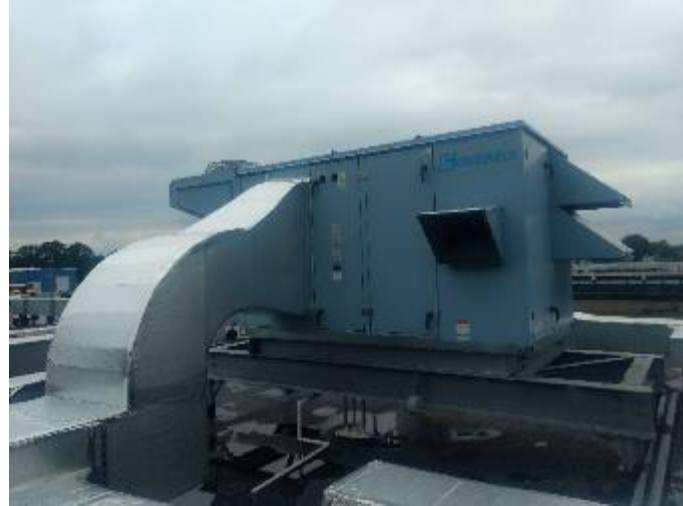
Fig 7b – A-Wing: Heat Pump HRV-1 (Greenheck ERCH)
