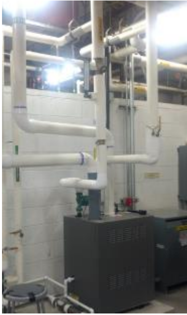
Fig 4a – Laars boiler
