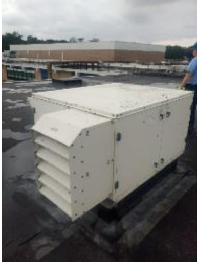
Fig 7a – E-Wing HRV (Greenheck)
