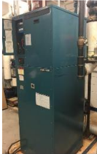
Image 5. Picture of the boilers
