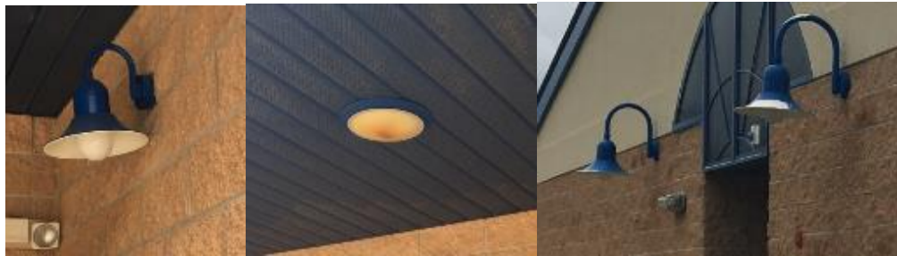
Image 4. Pictures of the various exterior HID lighting
