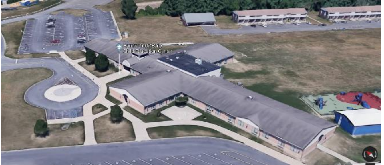
Image 1. Aerial screenshot of the building
