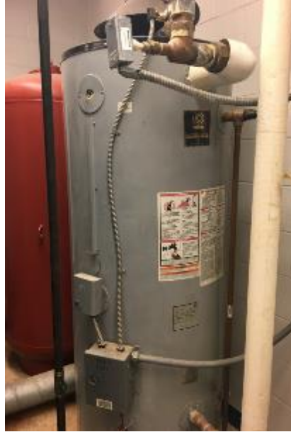
Image 7. Picture of the domestic hot water heater
