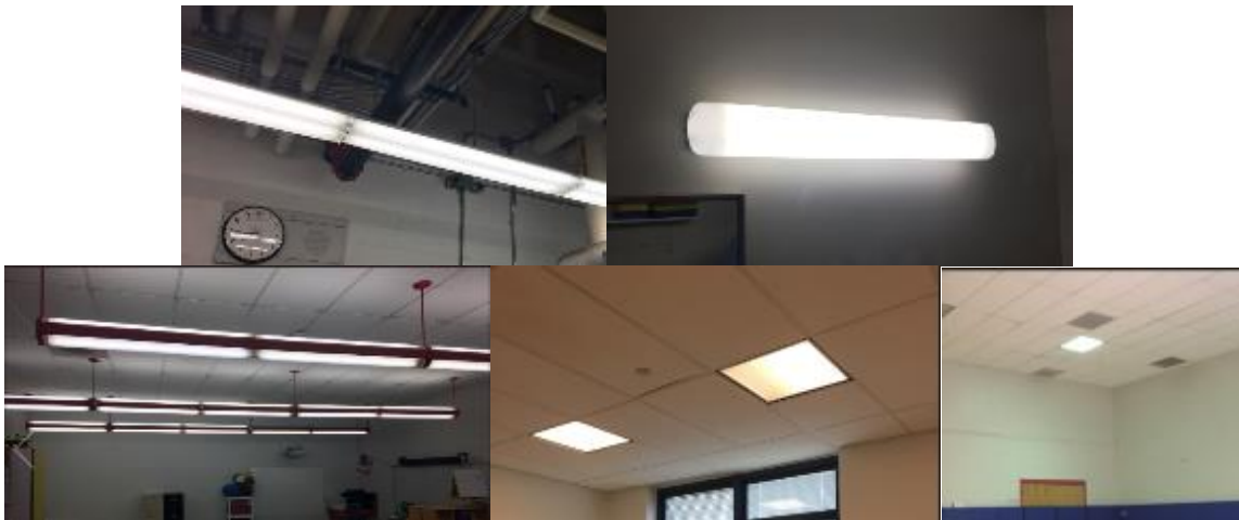
Image 2. Pictures of various fluorescent & HID interior lighting throughout the building
