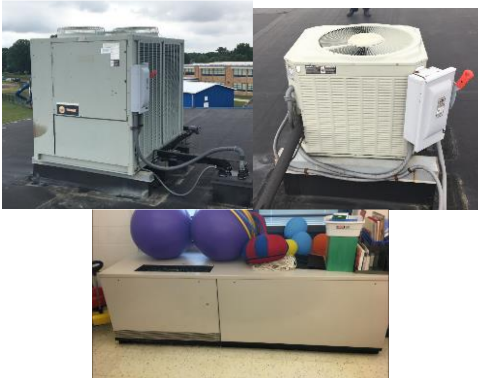
Image 6. Pictures of the condensing units of the air conditioning units and unit ventilator
