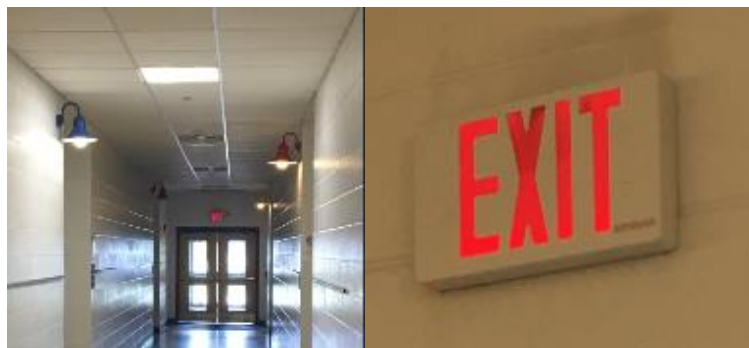
Image 3. Picture of hallway lighting and exit signs
