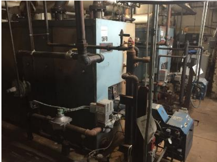
Figure 10 - Picture of the steam boiler
