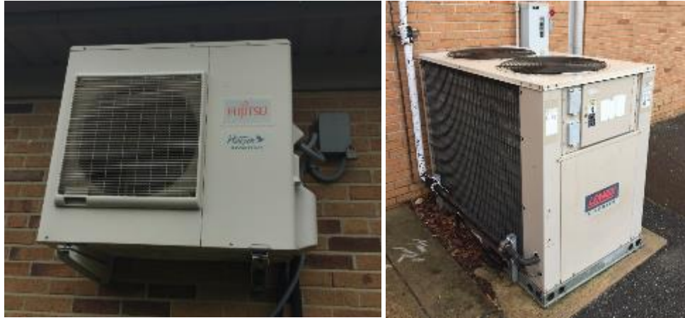
Figure 11 - Pictures of some of the condenser units of heat pumps and air conditioning units
