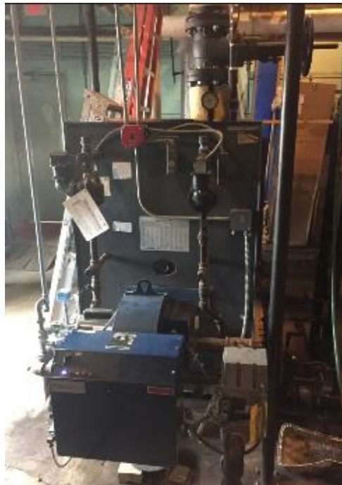
Figure 9 - Picture of the hot water boiler
