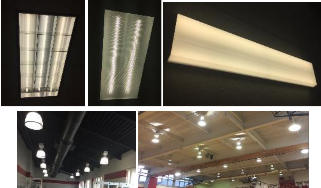
Figure 7 - Pictures of various fluorescent & HID interior lighting throughout the building
