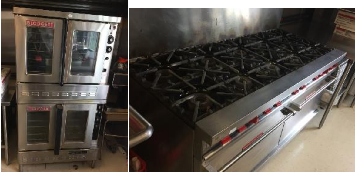
Figure 13 - Pictures of the gas cooking line and ovens
