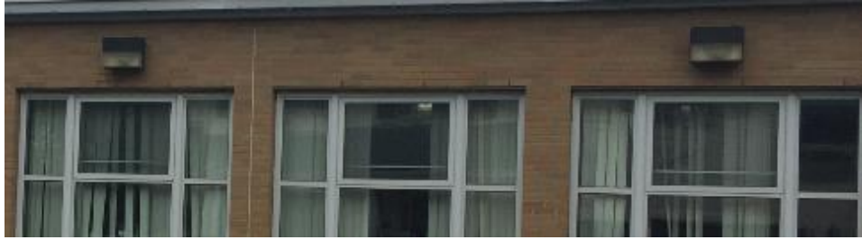
Figure 8 - Pictures of the various exterior HID lighting
