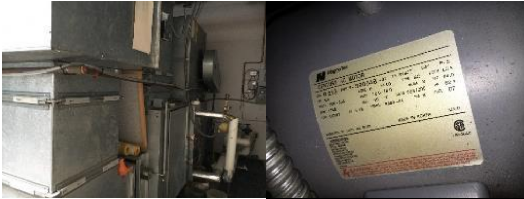
Library HVAC System and Supply Fan Motor Nameplate
