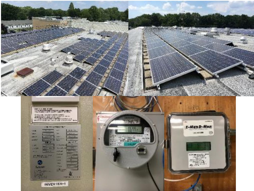
Roof Mounted Photovoltaic (PV) System
