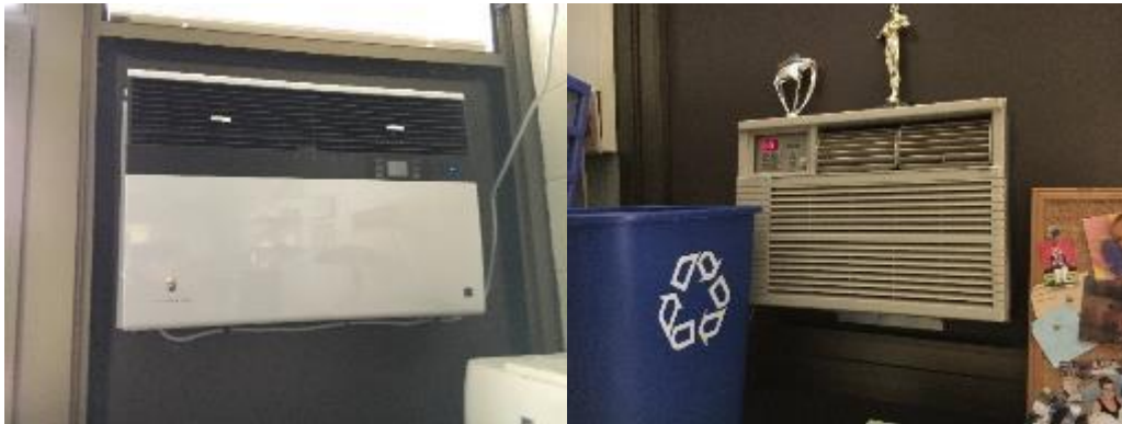
Window AC Units
