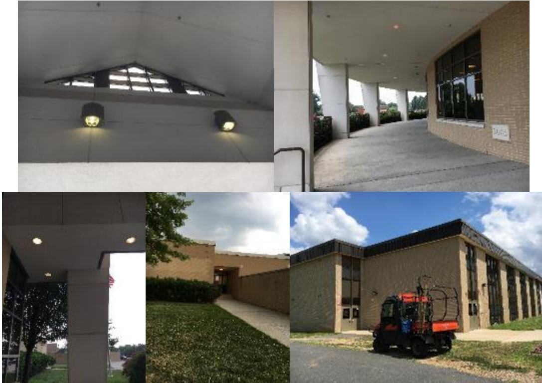
Exterior Lighting Systems
