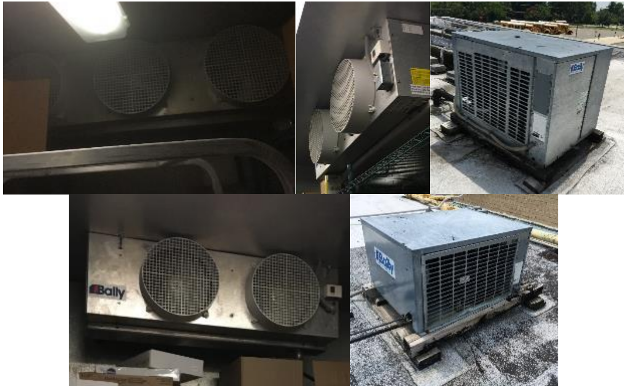
Walk in Refrigeration Equipment
