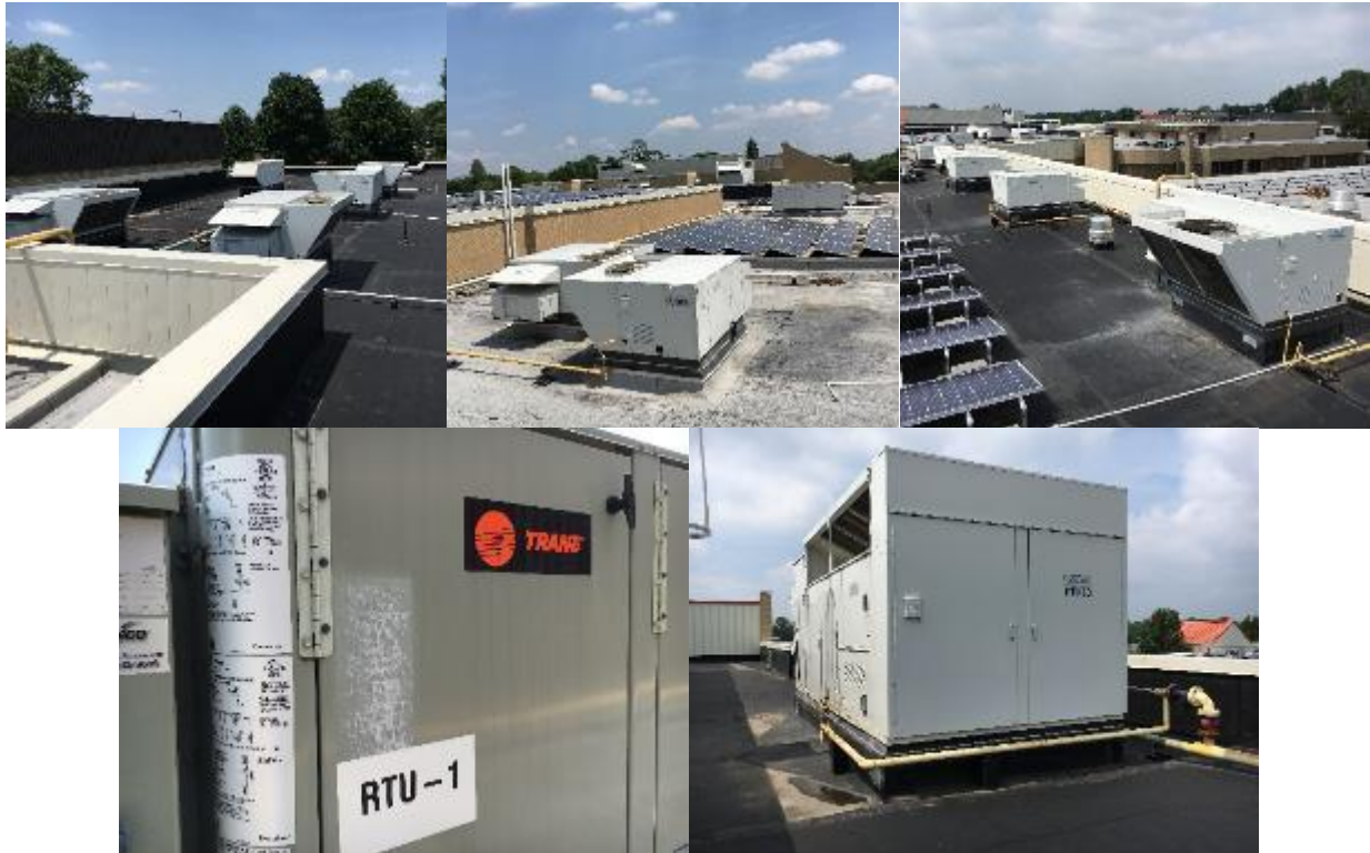
Typical Roof Top Units (RTUs)
