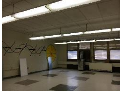
Old T8 4 Wrap Fixtures in Continuous Rows to be Replaced by New LED Panels
