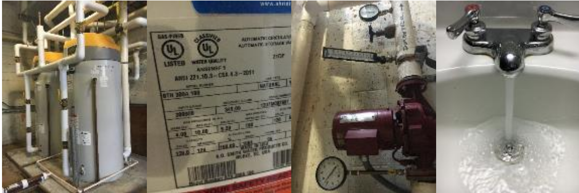
Domestic Hot Water Heating System
