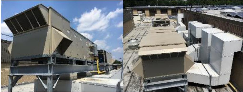
Gymnasium Energy Recovery Units (ERUs)
