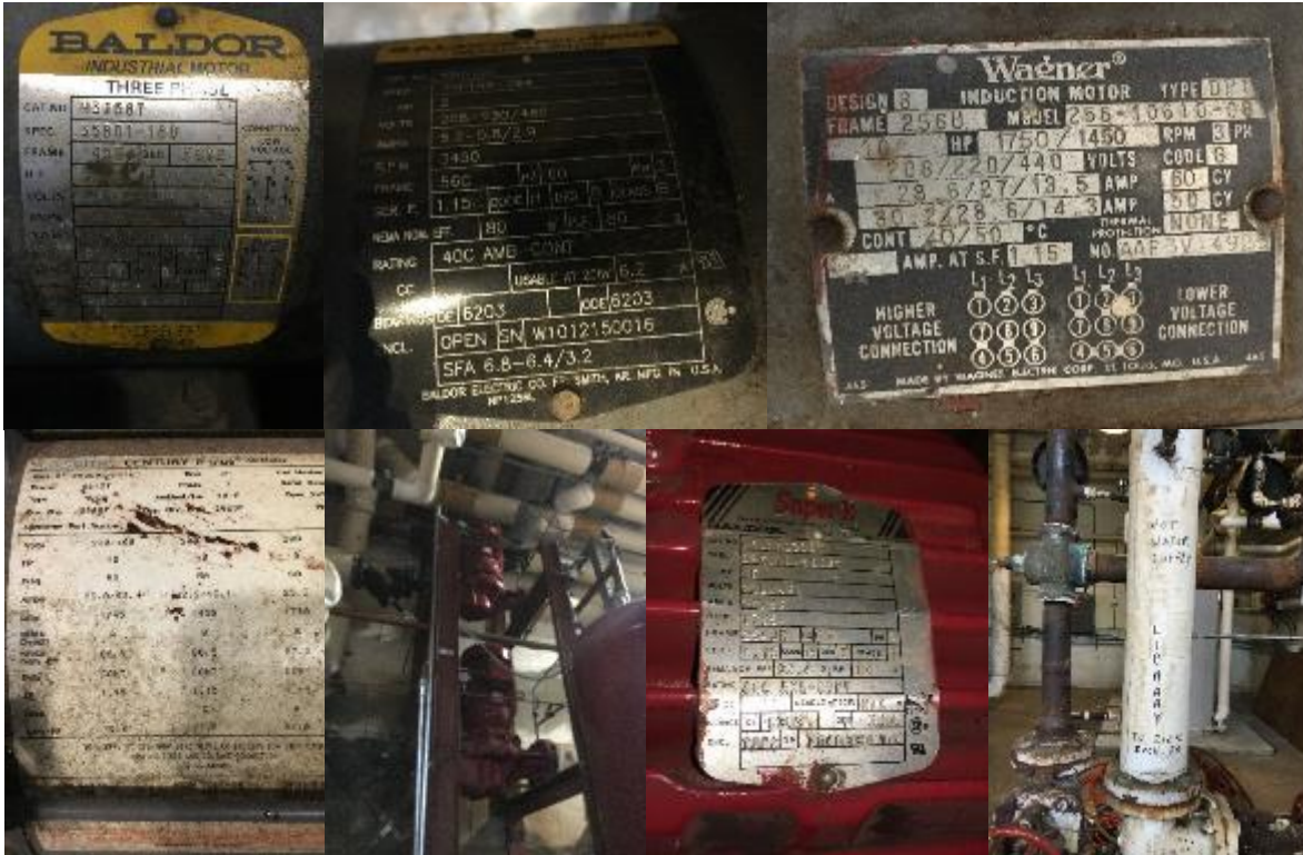
Boiler Burner Motors and Hot Water Pump Motors
