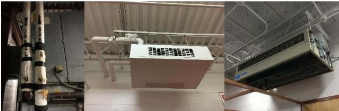
Gymnasium and Locker Room Heating-Ventilating (HV) Units with Hot Water Coils
