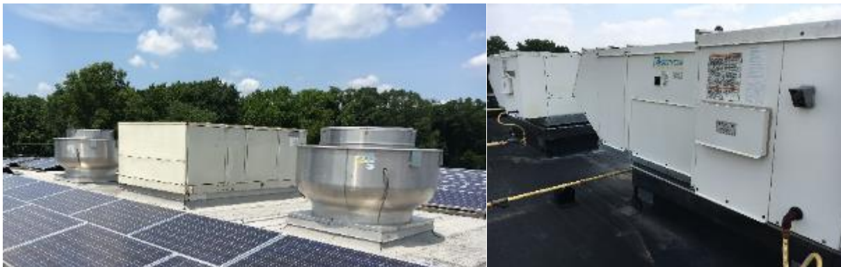
Pool Heating and Ventilation System and Make Up Air Units (MUAs)
