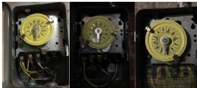
Exterior Lighting Timeclock Controls
