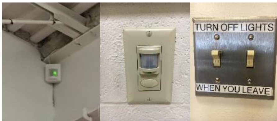
Interior Lighting Controls
