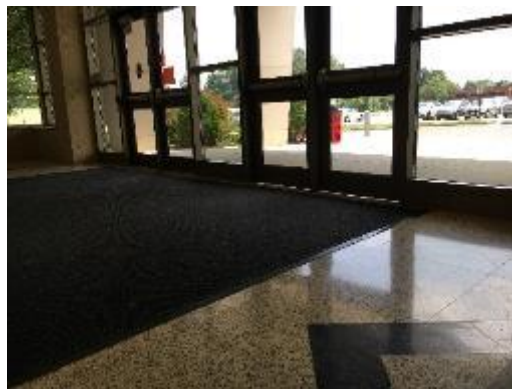
Building Envelope Deficiencies
