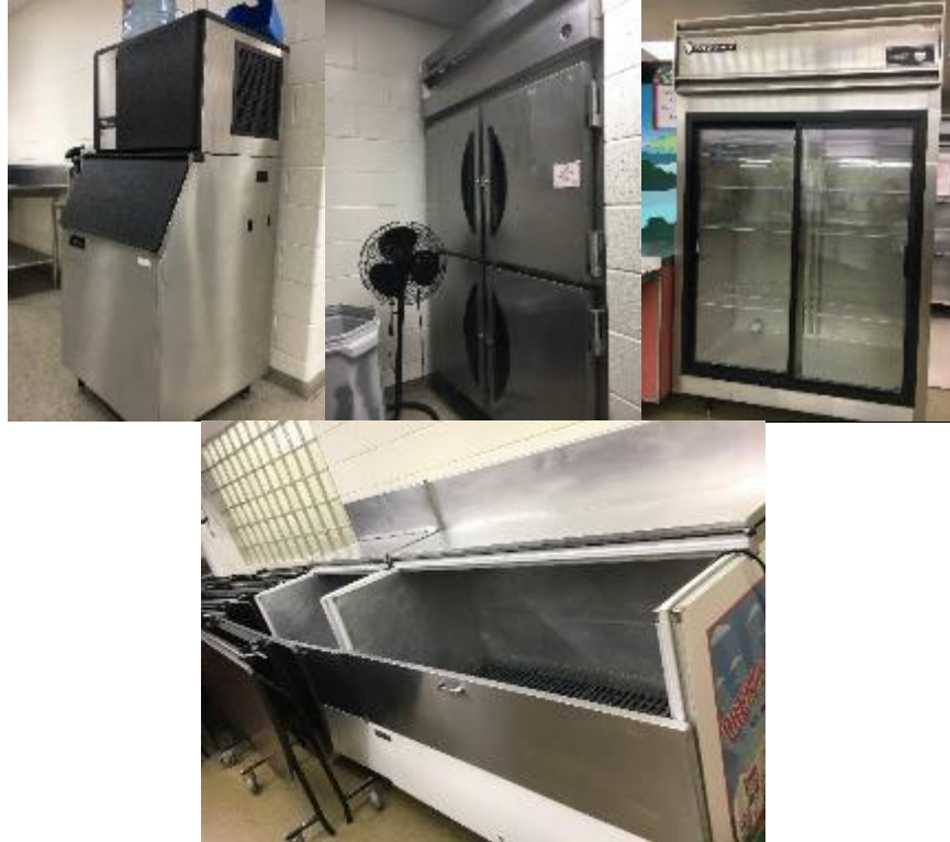
Ice Maker and Stand-up Refrigeration Equipment
