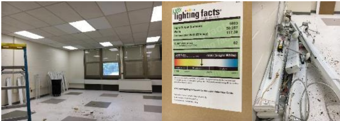
New LED Lay-in 2x4 Panel under construction in 2 nd floor classroom
