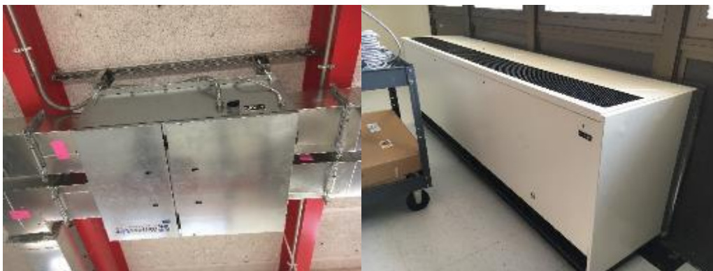
Athletics Room Energy Recovery Ventilator (ERV) and Classroom Unit Ventilator
