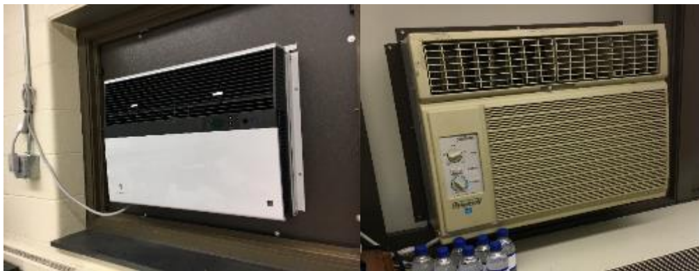
Window AC Units
