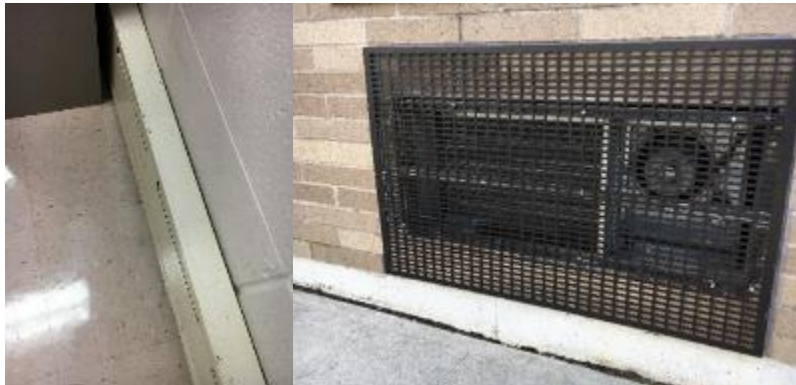
Baseboard Radiators and Unit Ventilators
