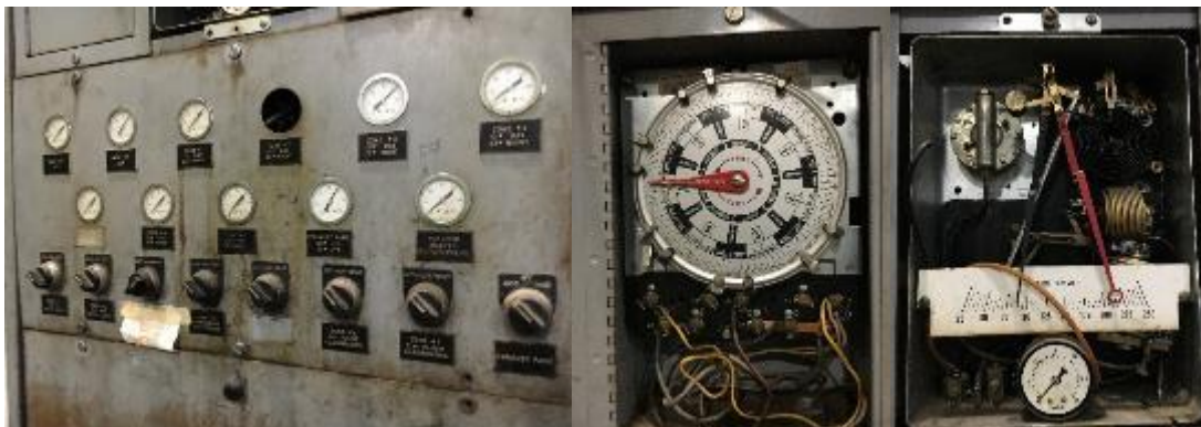
Original Heating and Ventilating (HV) Unit and Exhaust Fan Controls
