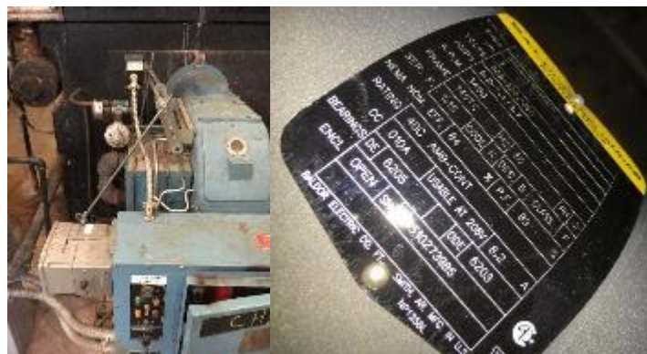
Boiler Burner Mechanical Linkage Type and Motor
