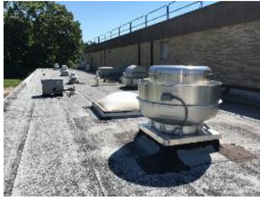
Kitchen Exhaust and Walk-in Cooler Outdoor Condensing Unit
