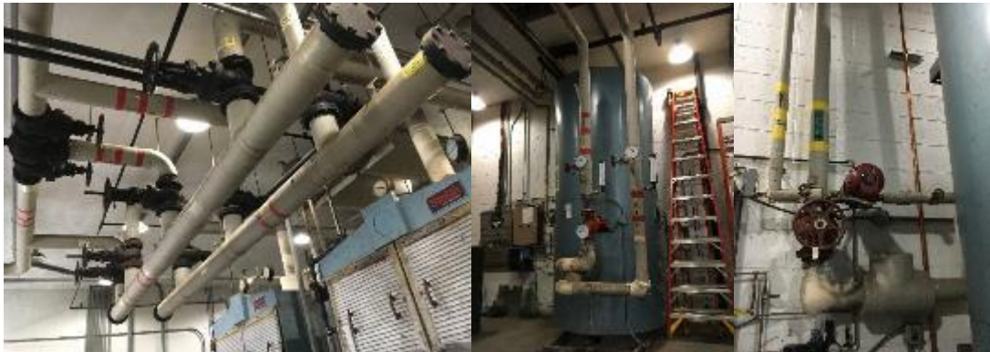
Heat Exchanger and Domestic Hot Water Storage Tank and System
