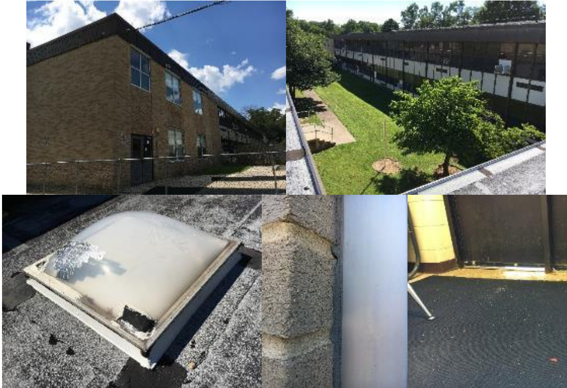
Building Envelope Deficiencies
