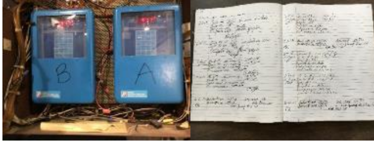
Boiler Controls and Winter Boiler Status Notes
