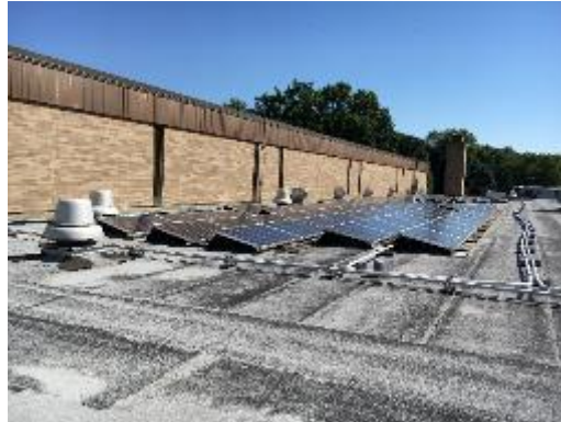
Roof Mounted Photovoltaic (PV) System
