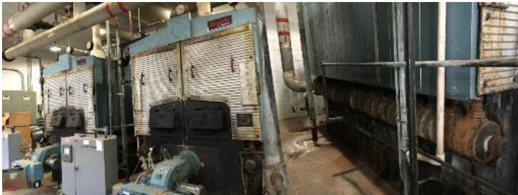
Cast Iron Boilers in Poor Condition
