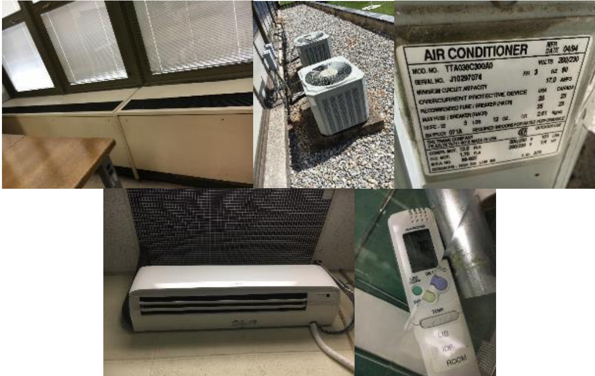
Split Air-Conditioning (AC) Systems
