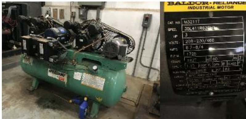
Air Compressor for Pneumatic HVAC Controls
