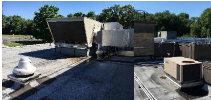
Roof Top Units
