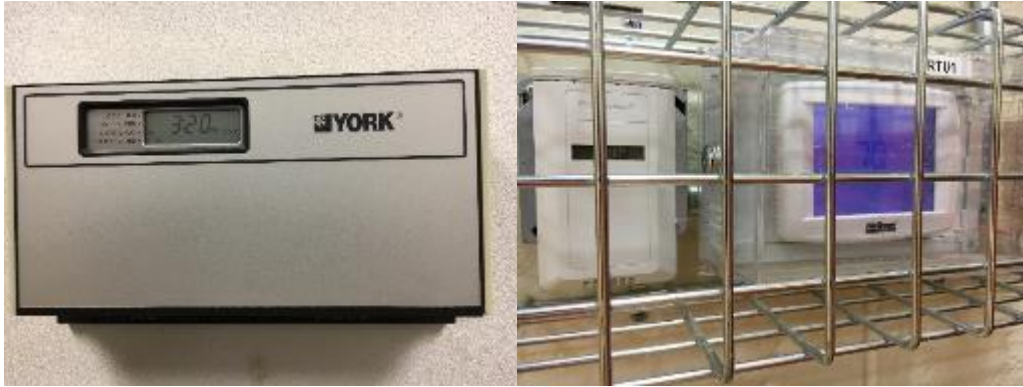
Programmable Thermostats for York RTU and Gym McQuay RTU
