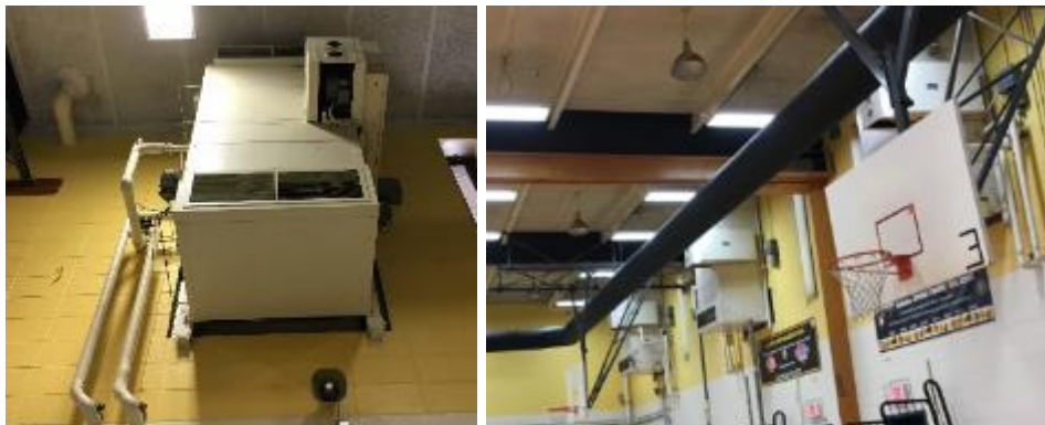
Heating and Ventilating (HV) Units in Gymnasium and Multi-Purpose Room
