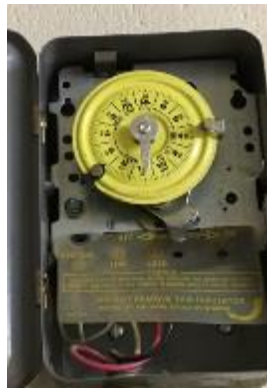
Exterior Timeclock Controls
