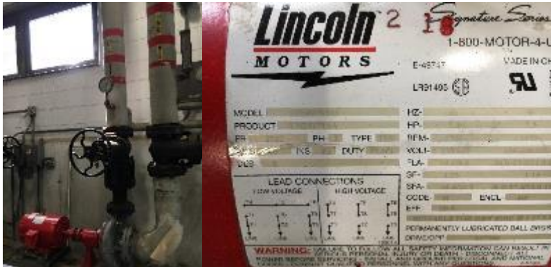
Hot Water Pumps and Motors
