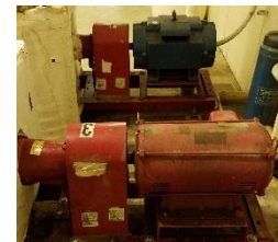
Figure 18 - Constant Speed 20 hp pumps
