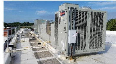
Figure 27 - 30-ton RTU with ERV - cafetorium
