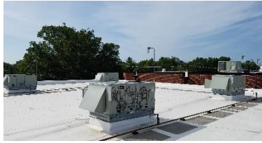
Figure 26 - 5-ton RTUs - new gym
