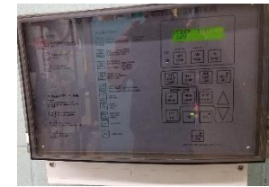
Figure 21 - Aerco control panel with OA reset function
