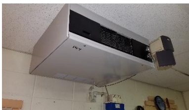
Figure 22 - Fan coil unit with condensate pump
