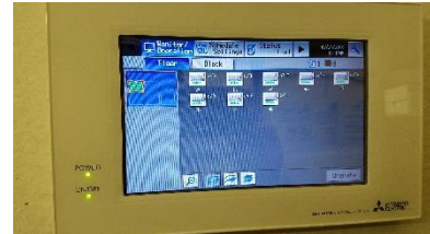
Figure 30 - Mitsubishi Multi City heat pump system control panel
