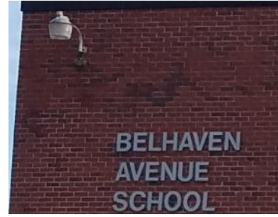
Figure 15 - Photo cell controlled area fixture
