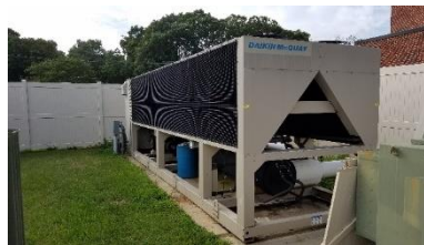
Figure 17 - McQuay air-cooled chiller
