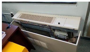
Figure 23 - Unit ventilator in an office
