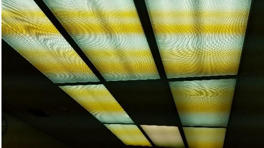
Figure 9 - 4-lamp T12 fixtures
