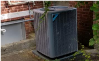
Figure 28 - Daikin split-system heat pump
