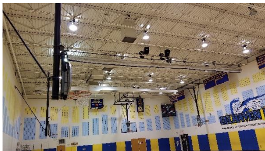
Figure 11 - Metal halide high bay fixtures in the gym
