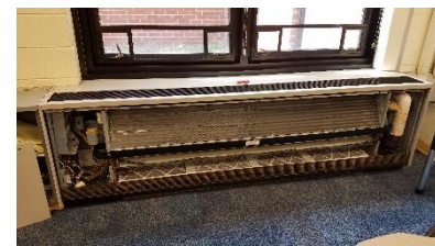
Figure 24 - Unit ventilator in a classroom
