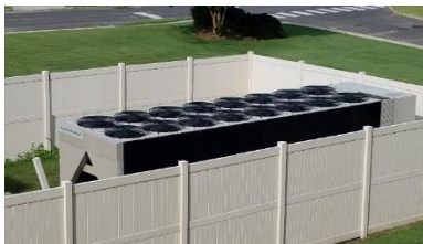
Figure 16 - McQuay air-cooled chiller
