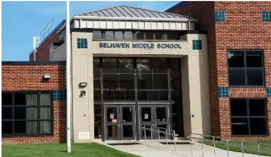
Figure 7 - Front entrance with aluminum and glass facade
