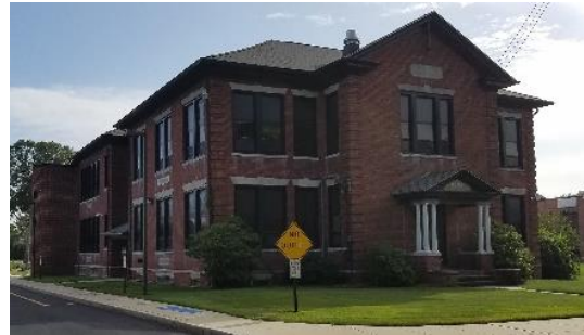
Figure 8 - 1908 - note replacement windows
