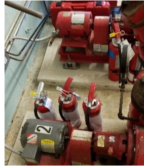
Figure 20 - Heating hot water pumps
