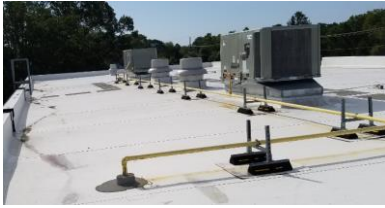
Figure 25 - 10-ton RTUs - new gym
