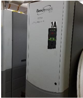
Figure 19 - Aerco Benchmark 2.0 high efficiency boiler
