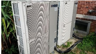
Figure 29 - Mitsubishi City Multi - multi-split ductless heat pumps
