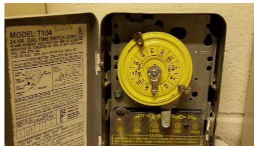
Figure 12 - Exterior fixture timer
