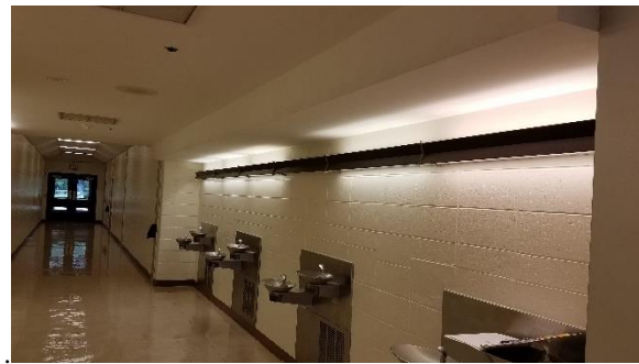
Figure 10 – Indirect lighting in the north corridor
