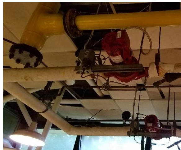
Figure 14 – Heating hot water circulating pumps
