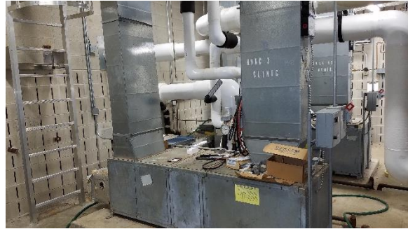
Figure 16 – AHUs "HVAC 3" and "HVAC 4"
