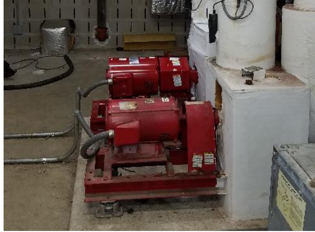
Figure 12 – 15 hp Chilled water pump
