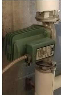
Figure 20 – Domestic Hot Water Circulator
