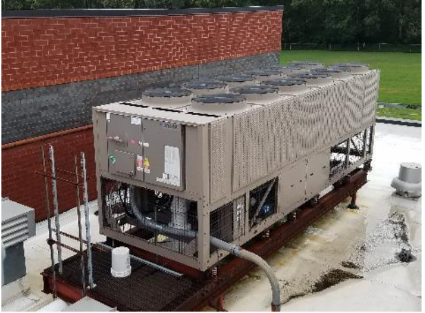
Figure 11 – York air cooled chiller
