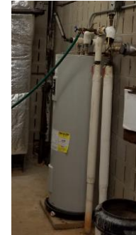
Figure 21 – Electric Domestic Hot Water Heater
