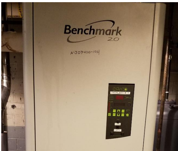
Figure 13 – Aerco high efficiency boiler
