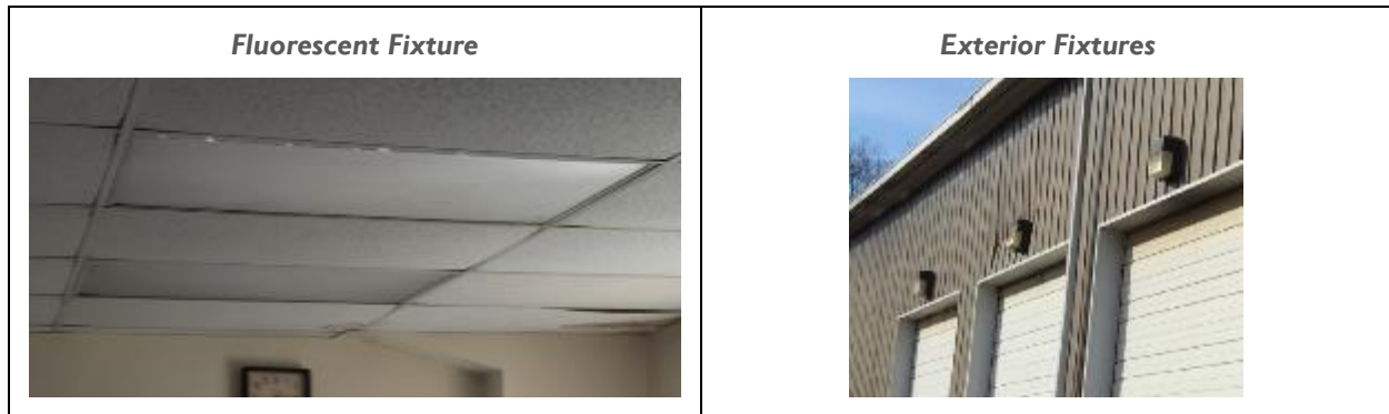
Figure 7 - Building Lighting Systems
