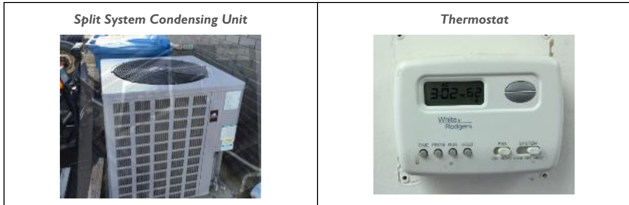
Figure 9 - Building AC Systems
