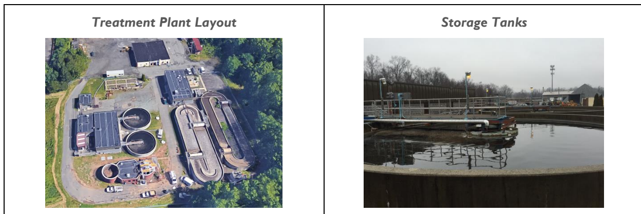
Figure 12 – Sewage Treatment Plant
