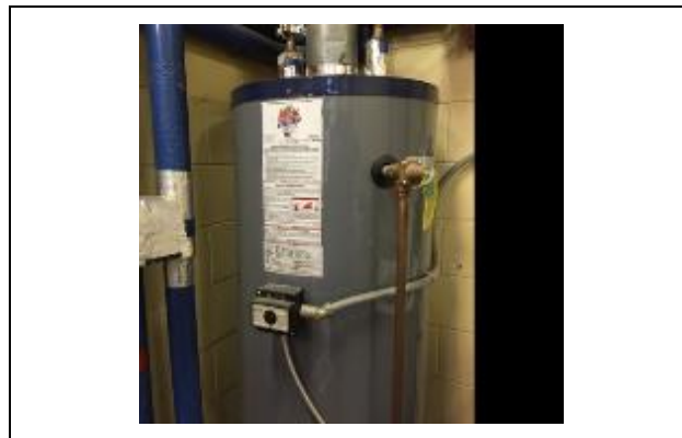
Figure 11 – Domestic Hot Water Heater
