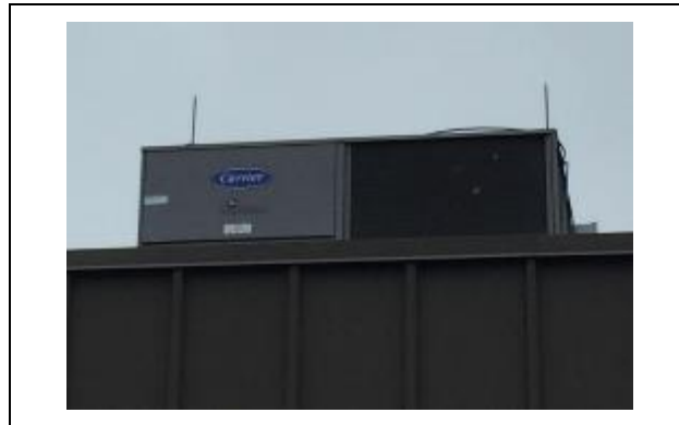
Figure 10 – Rooftop Package Unit
