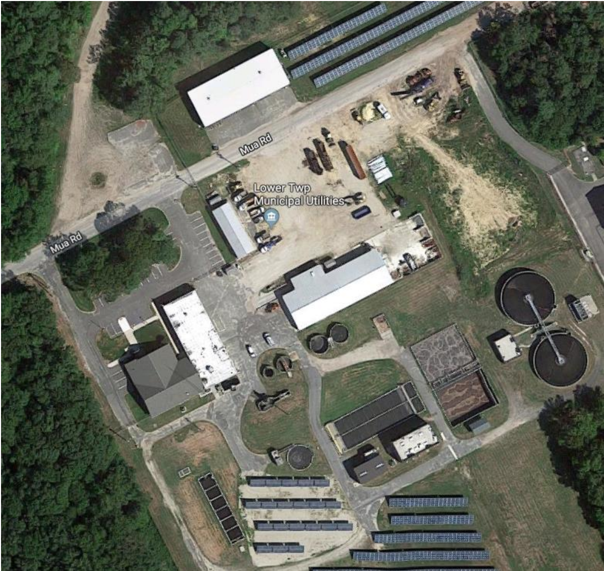
Image 1: Wastewater Treatment Plant Overview
