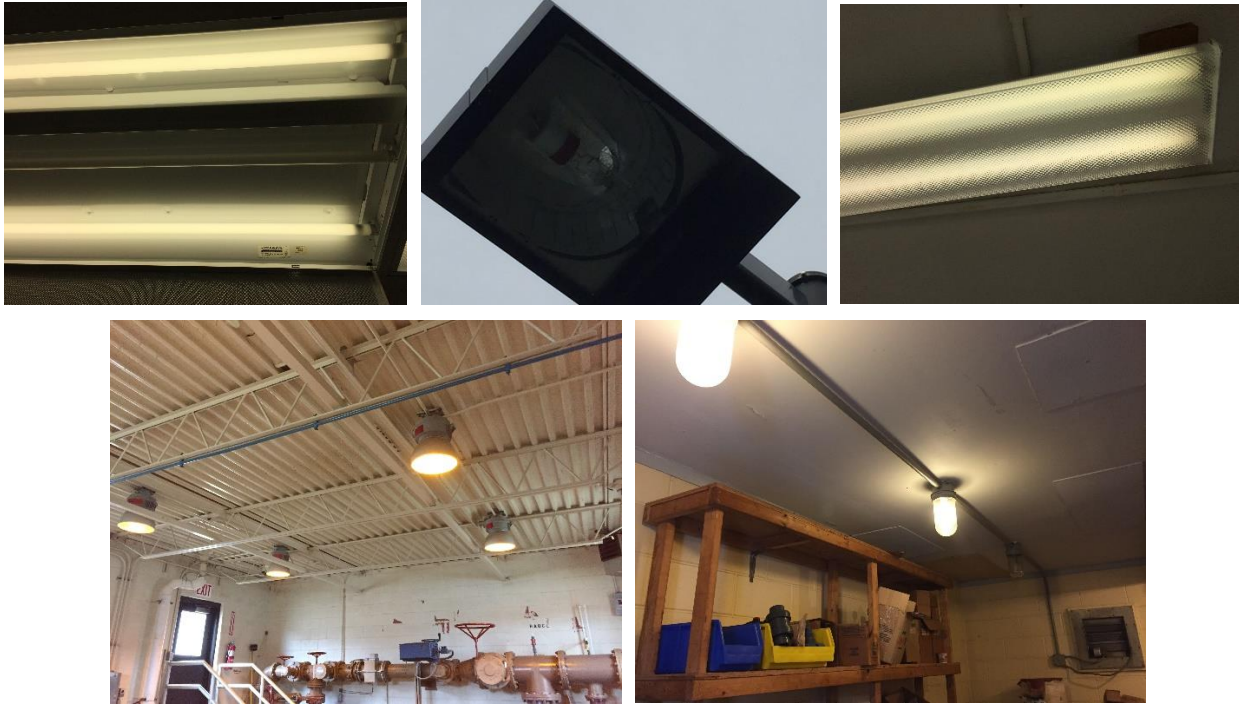
Image 2: Various Light Fixtures at the Facility
