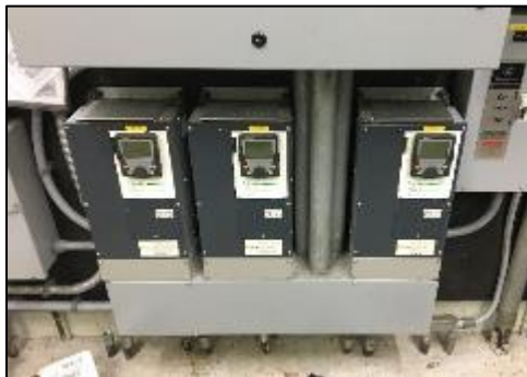
Image 6, 7 - VFDs, Electric Heater
