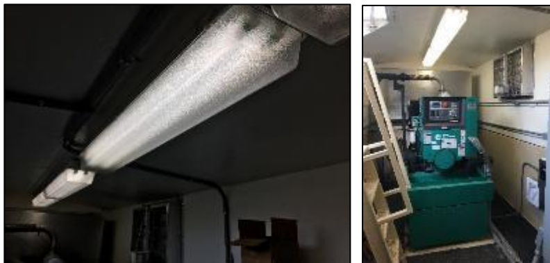
Image 19, 20 – Interior Lighting, Generator
