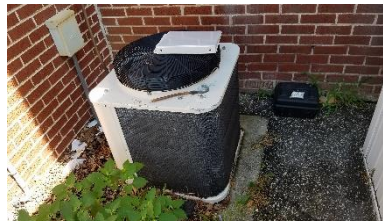
Figure 15 - Ground mounted condenser
