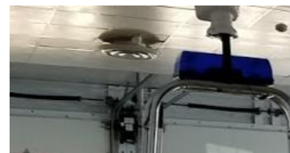
Figure 13 - Ceiling mounted fan coil unit in police garage
