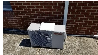
Figure 16 - Mini-split heat pump condenser
