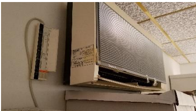
Figure 17 - Minisplit indoor unit (condenser on the roof)
