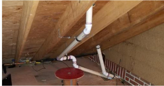
Figure 20 - Condensing furnace intake and exhaust piping
