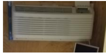
Figure 19 - PTAC in IT room.
