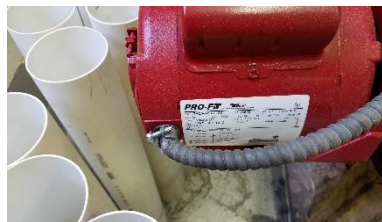
Figure 9 - Heating hot water circulator
