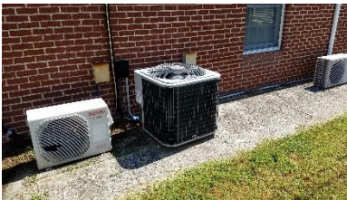
Figure 14 - Ground mounted condensers
