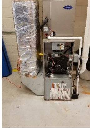
Figure 12 - Carrier 58MXA040 Furnace
