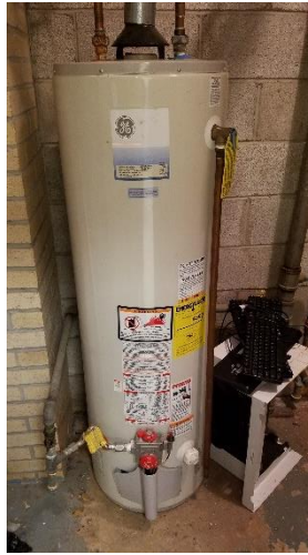
Figure 15 - GE 40-Gallon Hot Water Heater
