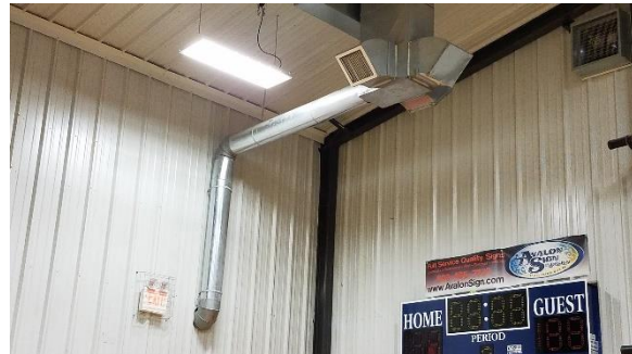
Figure 14 - Roof Top Unit Supply Terminus with duct to Front Hallway (Alley)
