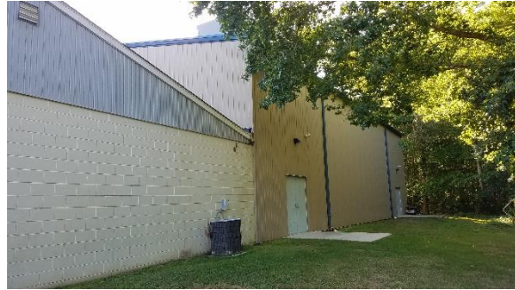
Figure 8 - Rear of Building
