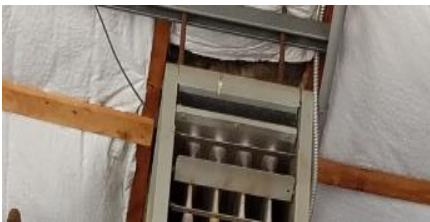
Figure 7 - Truck bay ceiling with gap in air barrier showing
