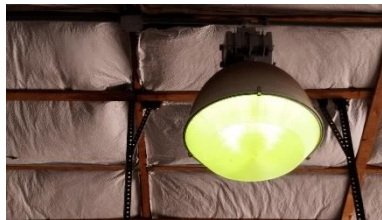
Figure 14 - Truck bay high bay metal halide fixture
