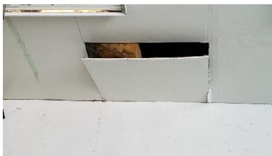
Figure 10 - Loose drywall in truck bay
