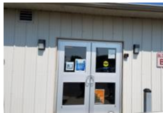
Figure 8 - Office building entrance
