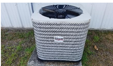
Figure 16 - Gibson 3.5-ton condenser
