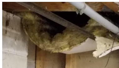
Figure 11 - Gap in air barrier in second story storage area.
