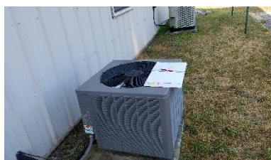
Figure 17 - Frigidaire 3-ton condenser
