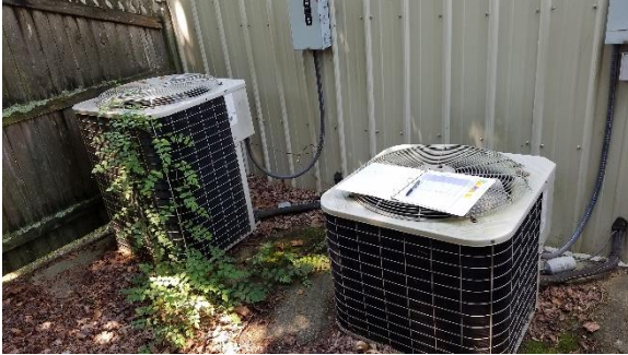
Figure 9 - 5-ton Outdoor Condensers
