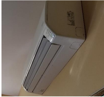
Figure 10 - Indoor Fan Coil
