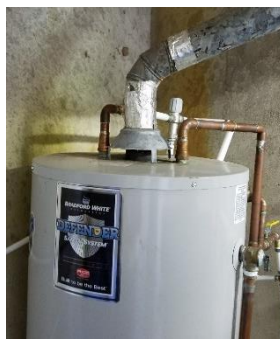
Figure 8 - Gas Fired DHW Heater
