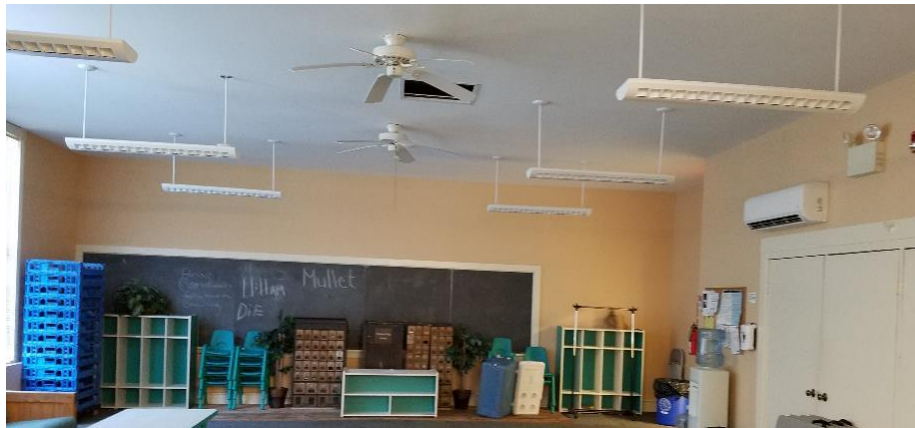
Figure 6 - Interior Linear Fluorescent Fixtures
