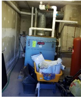
Figure 7 - Hot Water Heating Boiler
