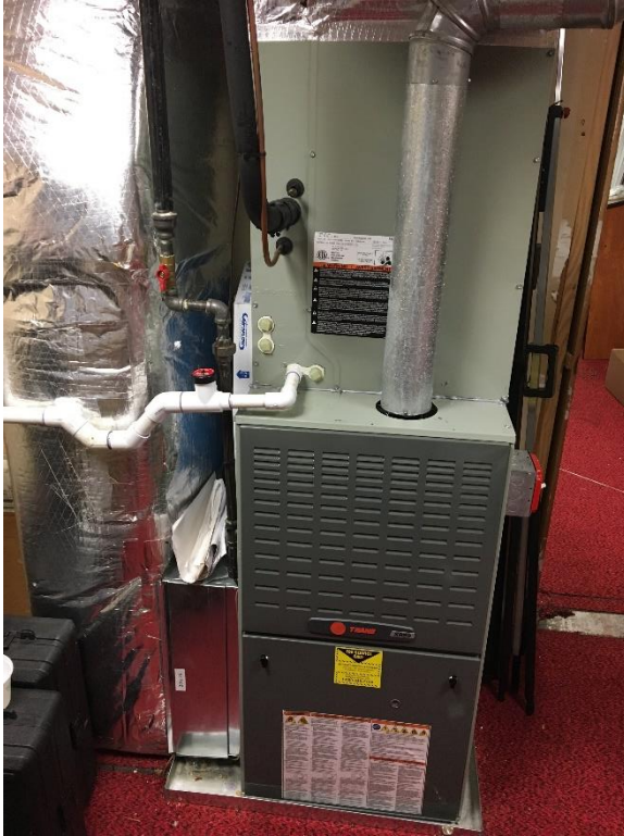
Image 9 – Trane XR80 AHU and furnace
