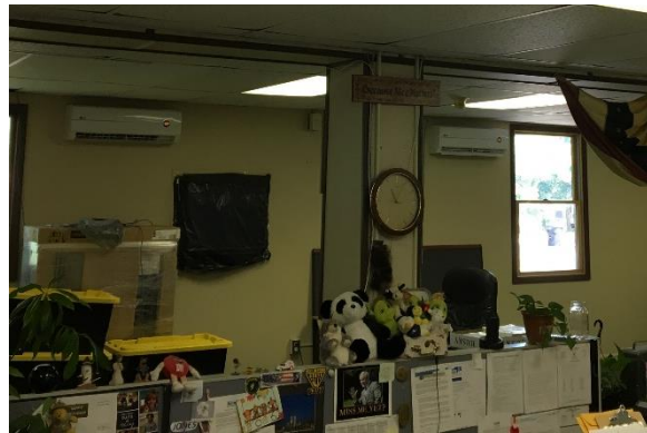
Image 8 – Indoor heat pump units
