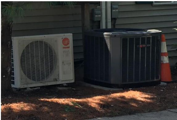
Image 7 – Outdoor heat pump unit & AC unit
