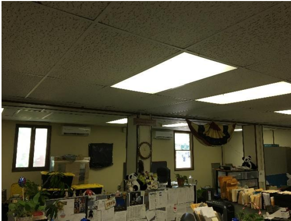
Image 5 – Typical linear fluorescent fixtures
