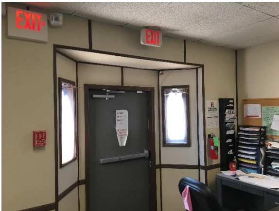
Image 3 – Typical exterior door
