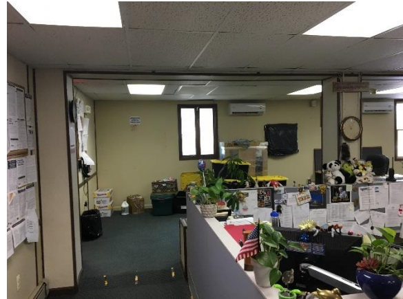
Image 6 – Typical linear fluorescent fixtures
