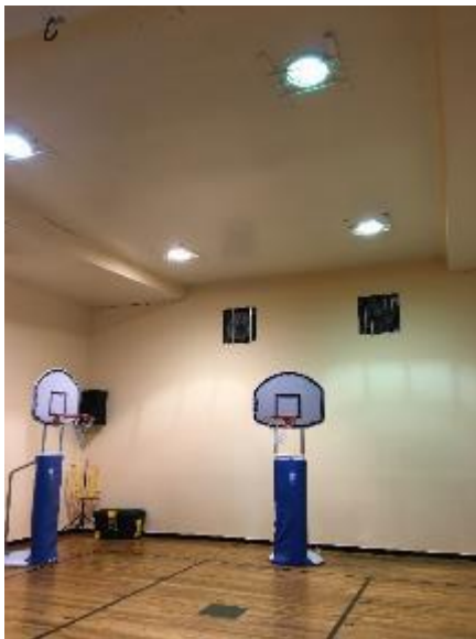
Image 7 – Gymnasium high bay fixtures
