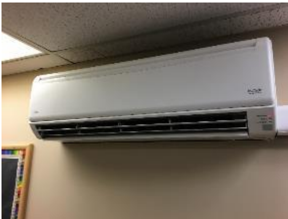
Image 13 – Fujitsu ductless mini-split system
