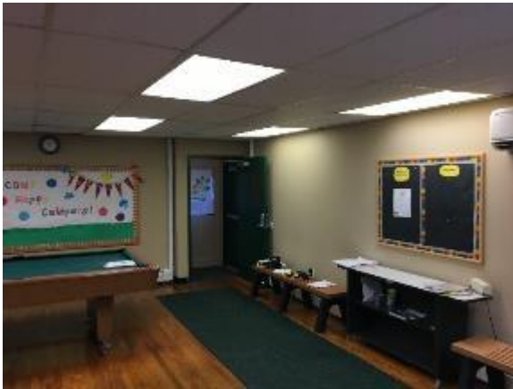
Image 5 – Typical linear fluorescent T8 lighting
