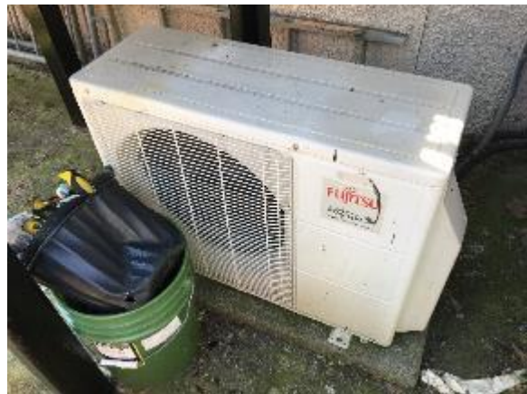
Image 14 – Fujitsu ductless mini-split system
