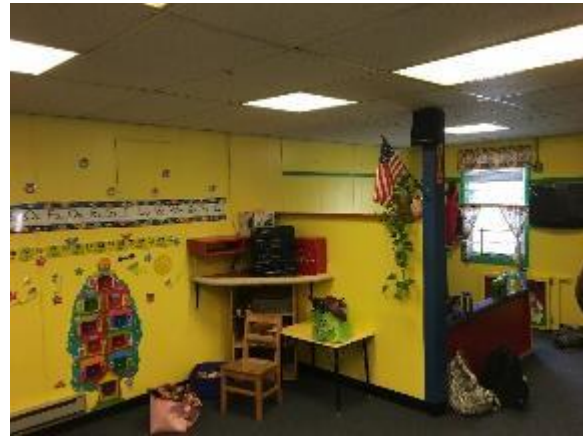
Image 6 – U-bend & 4 foot T8 fixtures
