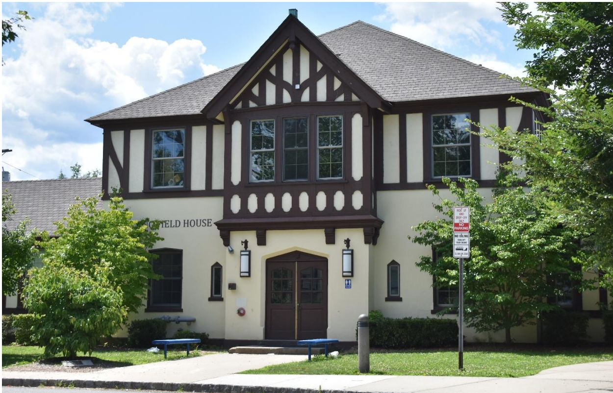
Image 1: Furlong Field House - Front Exterior
