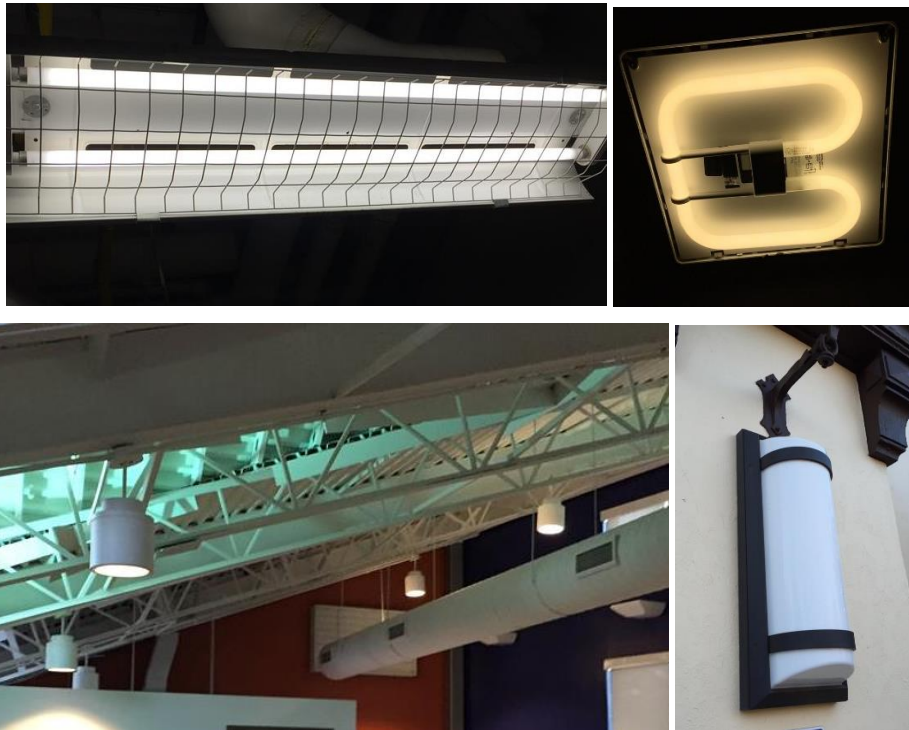
Image2: Furlong Field House / Woodman Field - Typical Lighting Fixtures
