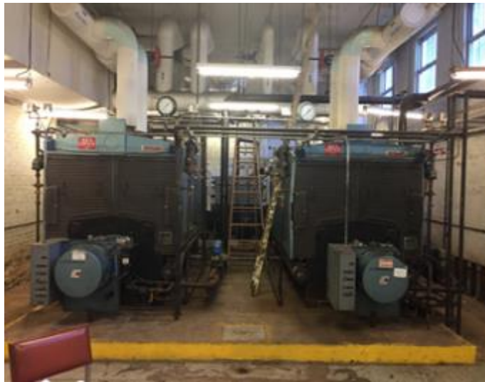
Image 3 – Steam Heating System (Boilers)
