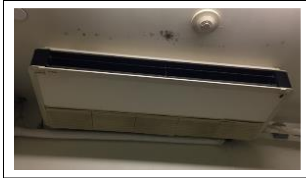
Figure 9 – DX Air Conditioning Systems
