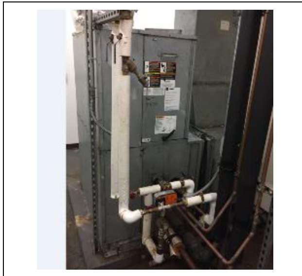
Figure 10 – Air Handling Unit
