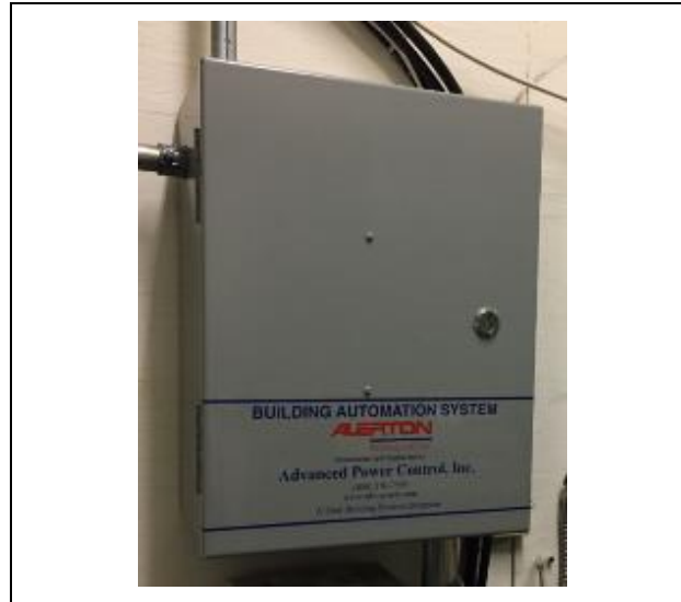
Figure 11 – Building Energy Management System Controller
