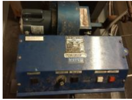
Hot Water Pumps
