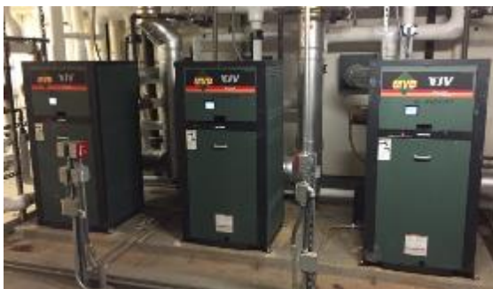
Domestic Hot Water Boilers
