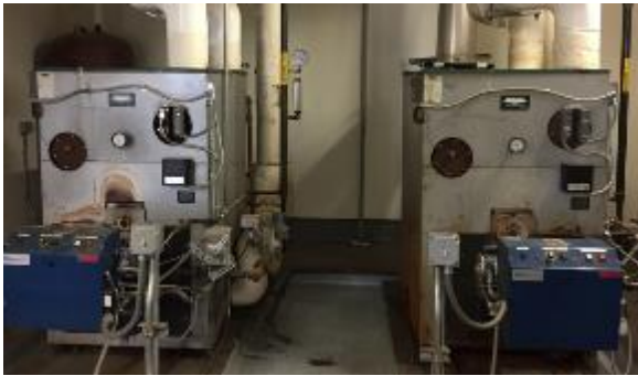
Heating Hot Water Boiler
