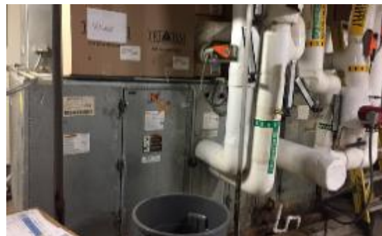
Air Handling Unit 2A
