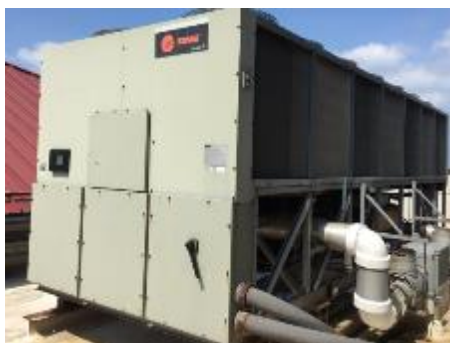
Air Cooled Chiller
