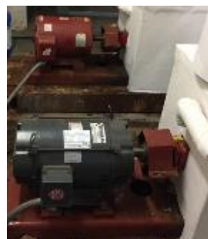
Chilled Water Pumps
