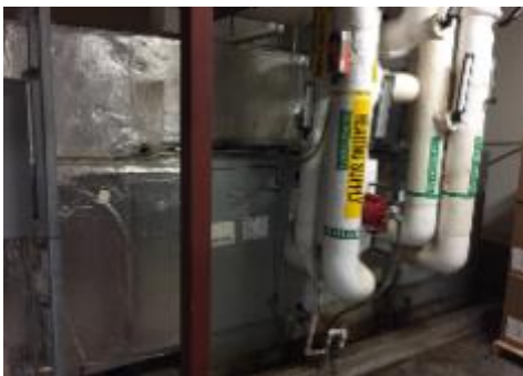
Air Handling Unit 1A
