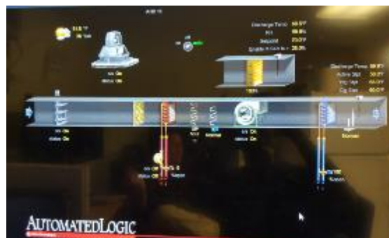
Air Handling EMS
