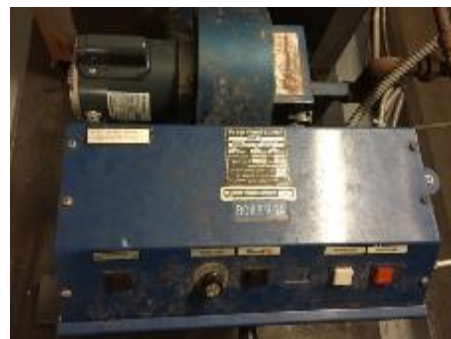
Hot Water Pumps
