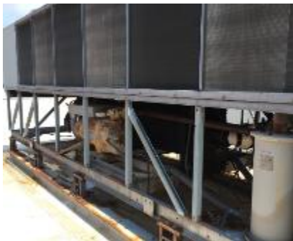
Air Cooled Chiller
