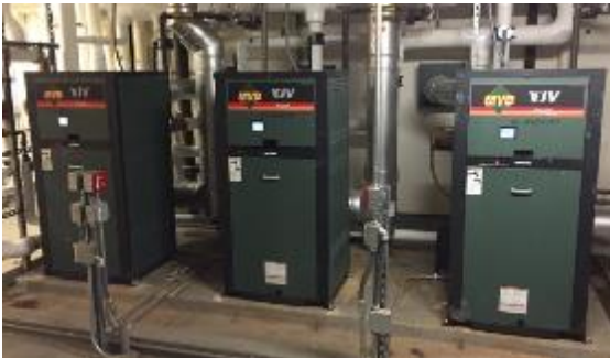
Domestic Hot Water Boilers
