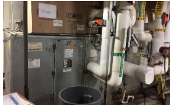
Air Handling Unit 2C
