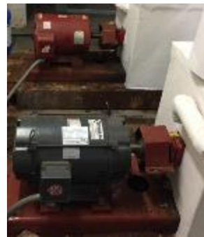
Chilled Water Pumps
