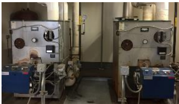
Heating Hot Water Boiler
