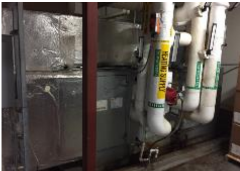
Air Handling Unit 1C
