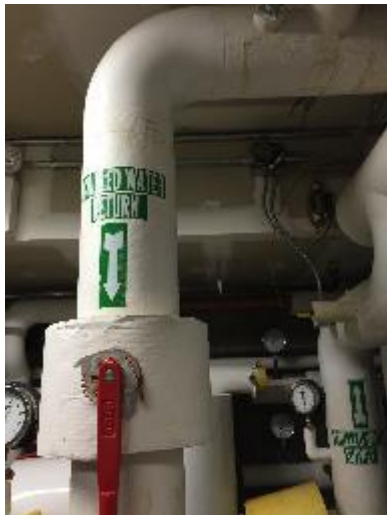
Image 3: Chilled Water System
