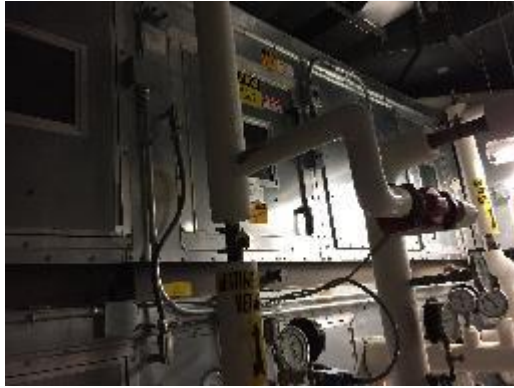
Image 5: Air Distribution System
