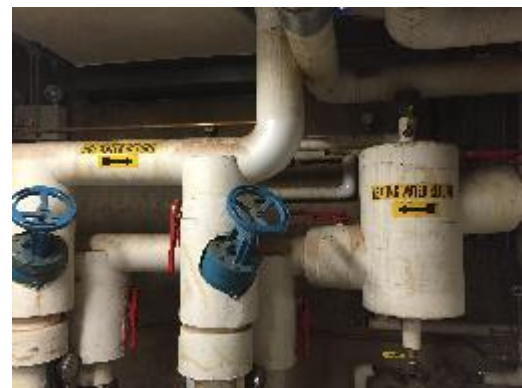
Image 4: Hot Water System
