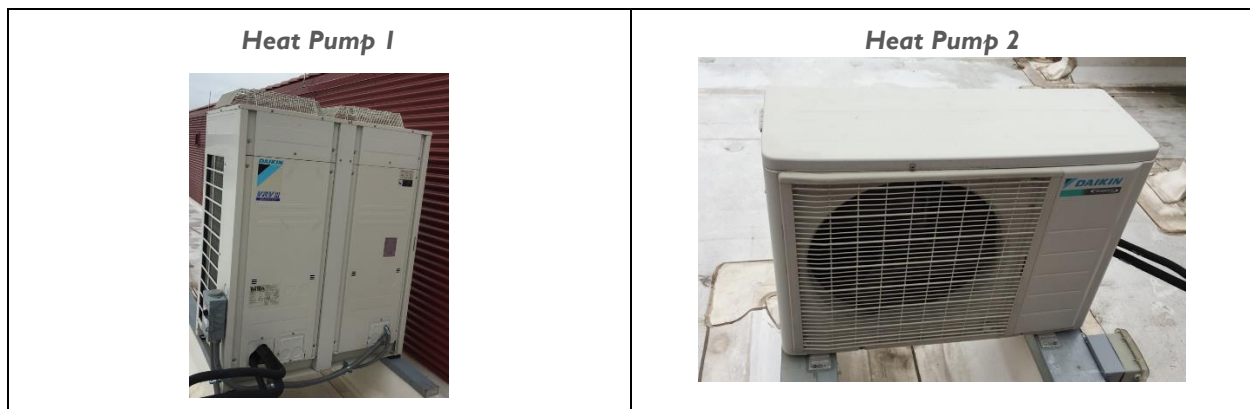
Figure 9 – DX Based Air Side Systems
