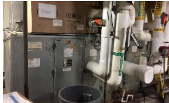
Air Handling Unit 2B
