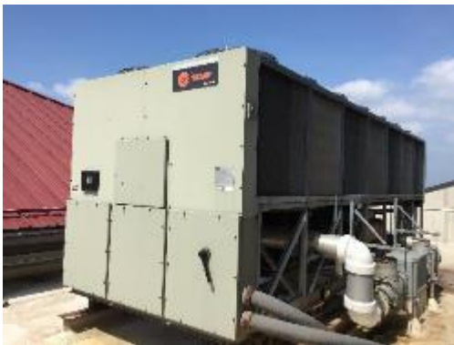
Air Cooled Chiller
