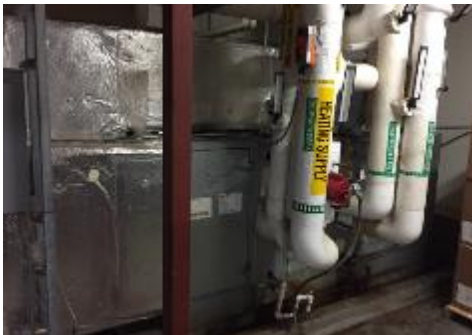
Air Handling Unit 1B
