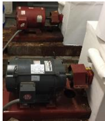
Chilled Water Pumps
