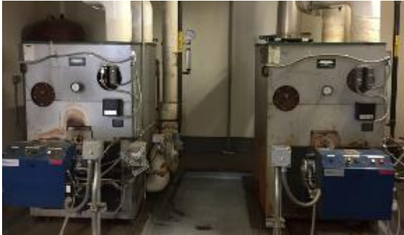
Heating Hot Water Boiler
