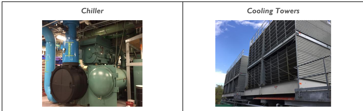
Figure 9 - Central Plant Equipment
