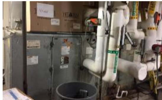
Air Handling Unit 2A
