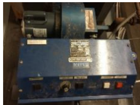
Hot Water Pumps
