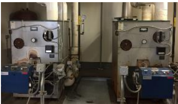
Heating Hot Water Boiler
