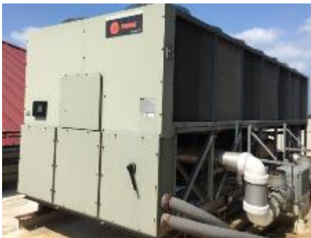
Air Cooled Chiller
