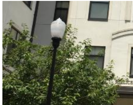
Exterior Pole Fixtures
