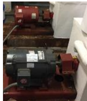
Chilled Water Pumps
