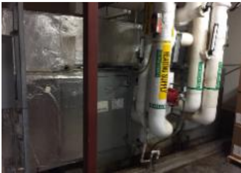
Air Handling Unit 1A
