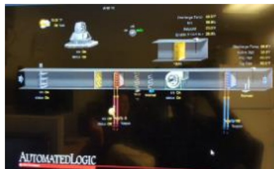
Air Handling EMS
