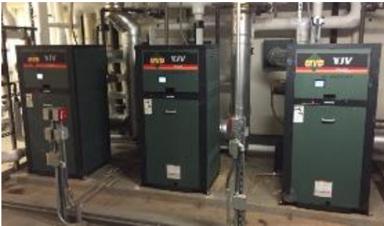
Domestic Hot Water Boilers
