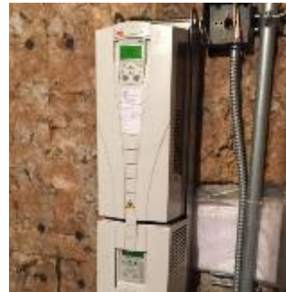
Typical Fan VFD
