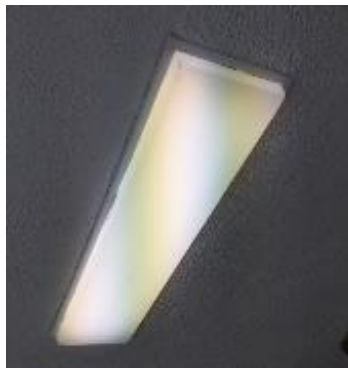
Typical Surface Mounted Fluorescent Fixture
