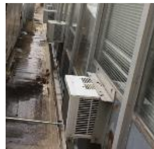
Window AC Units
