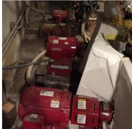
Figure 8 – Chilled Water Pumps
