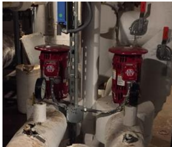
Figure 9 – Hot Water Pumps
