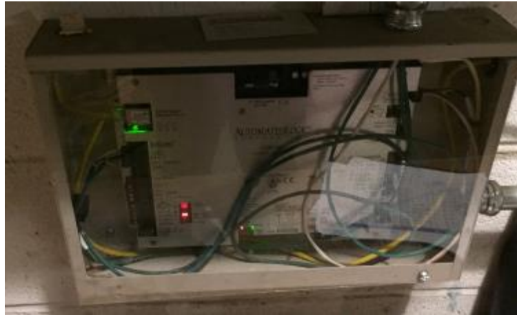
Figure 12 – Building Energy Management System Controller
