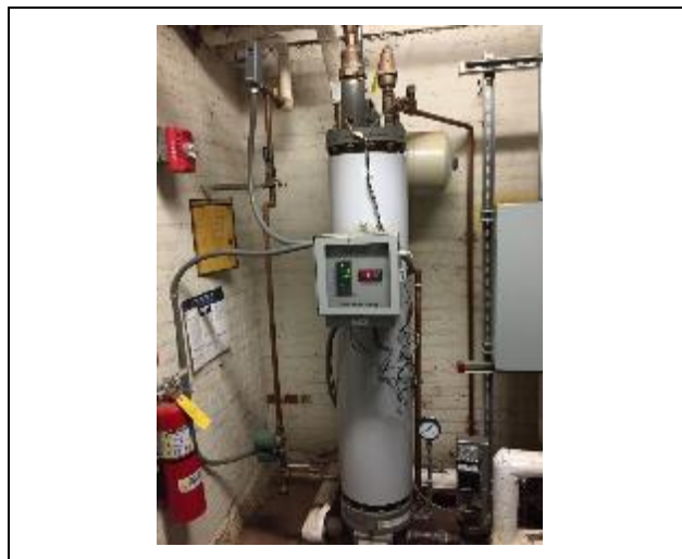
Figure 11 – Domestic Water Heater Exchanger
