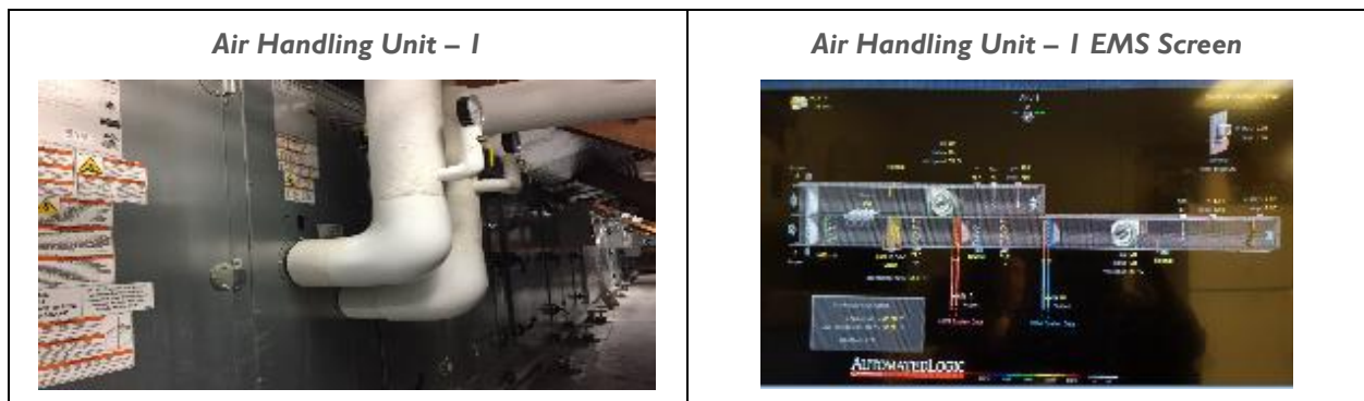
Figure 8 – Air Side Systems
