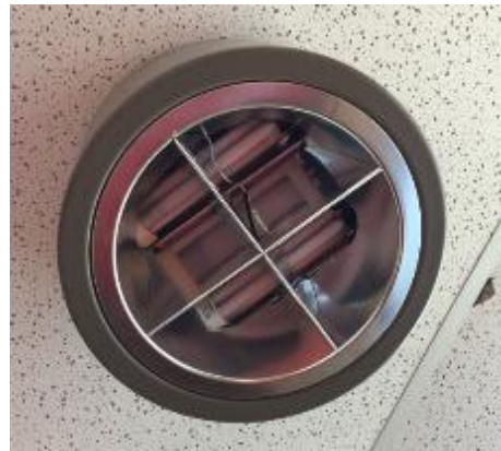
Typical Compact Fluorescent Fixture
