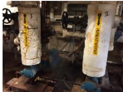
Hot Water Pumps
