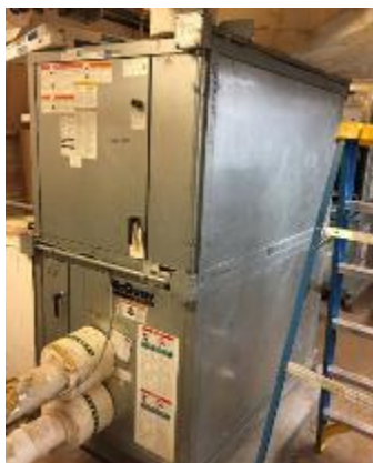
Air Handling Unit
