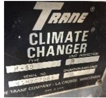
Air Handling Unit Nameplate
