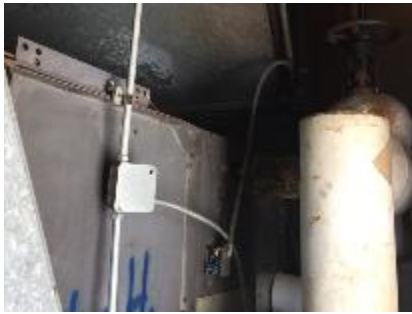
Air Handling Unit
