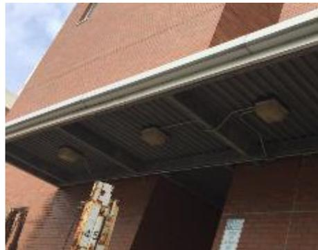
The building's exterior lighting consists primarily of inefficient 250-Watt and 400-Watt metal halide (MH) fixtures. In addition, there are some 250-Watt mercury vapor (MV) lamps that are controlled by DDC.
