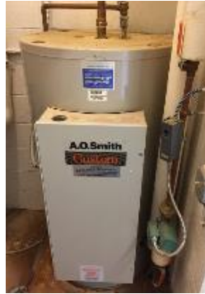
Figure 9 - Building Domestic Hot Water System
