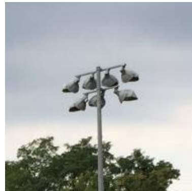
Typical Pole Mounted Fixture
