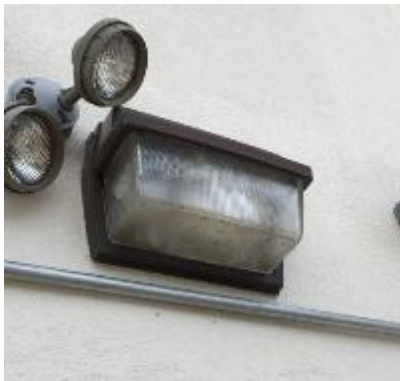
Typical Wall Mount Exterior Fixture
