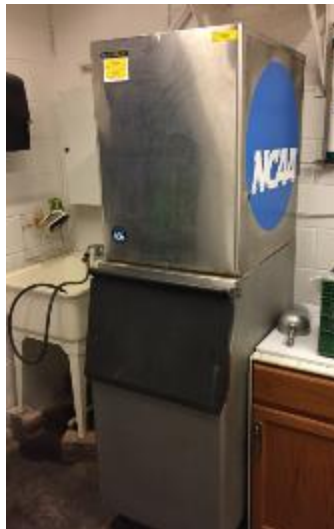
Figure 10 – Ice Making Equipment
