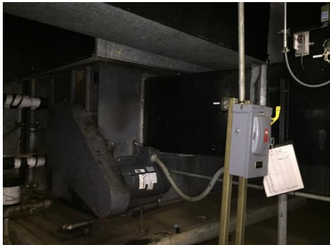
Air Handling Unit
