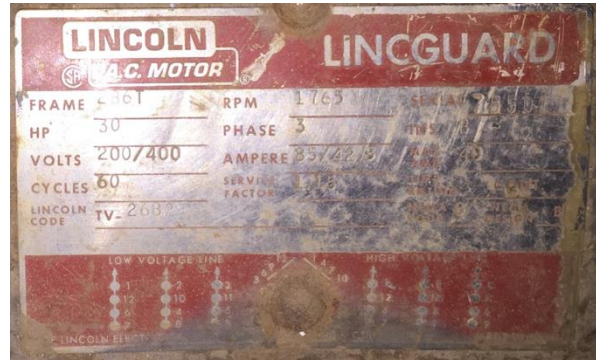
Chilled Water Pump Nameplate
