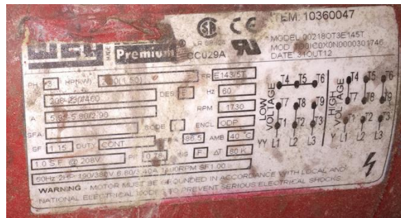
Hot Water Pump Nameplate
