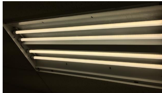
Typical T12 Fluorescent Fixture
