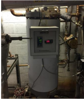
Steam to DHW Heat Exchanger
