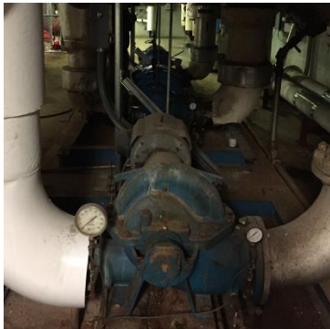
Chilled Water Pumps
