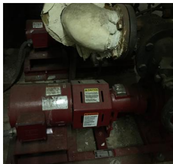
Hot Water Pumps
