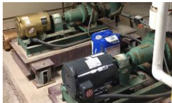
Hot Water Pumps
