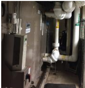
Air Handling Unit - 1
