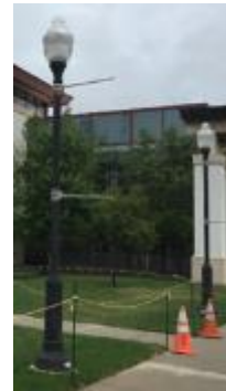
Exterior Pole Fixtures
