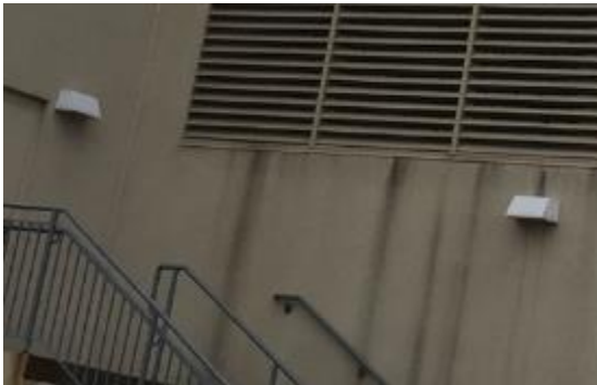
Typical Exterior Wallpacks
