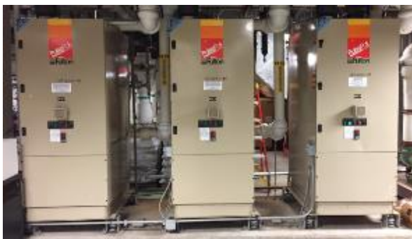
Heating Hot Water Boiler
