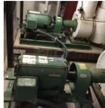
Chilled Water Pumps
