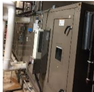
Air Handling Unit - 2
