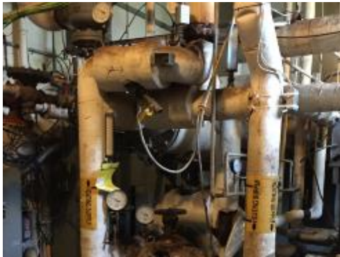
Steam to Hot Water HX
