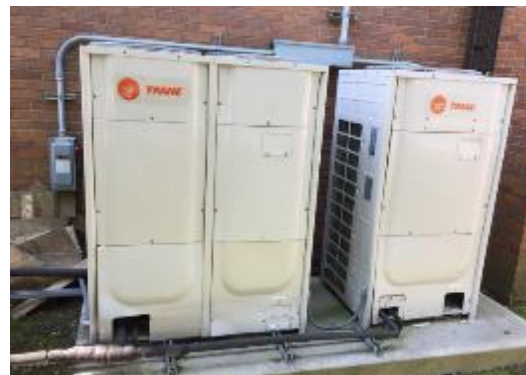
Split System Heat Pump
