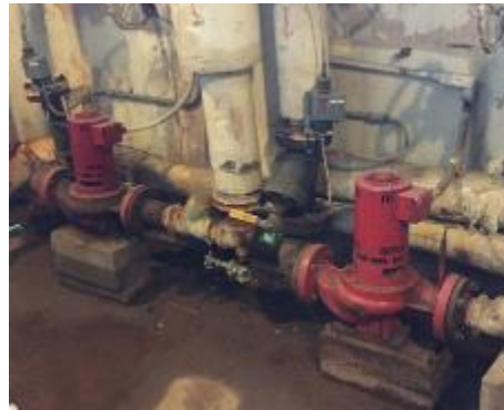
Hot Water Pumps
