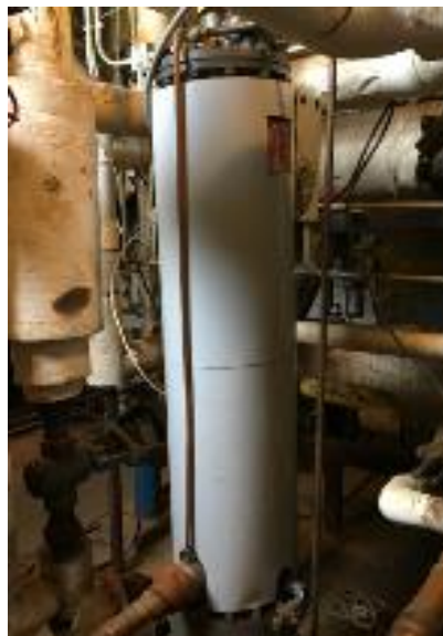
Steam to DHW Heat Exchanger
