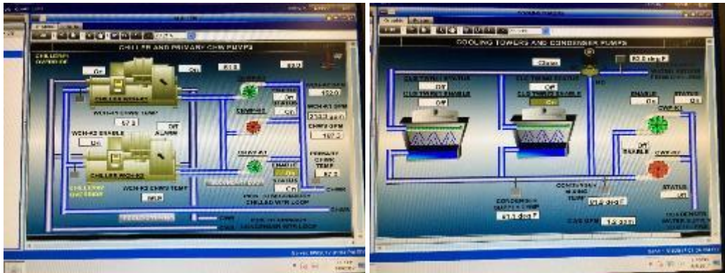
Cooling Controls, Energy Management System
