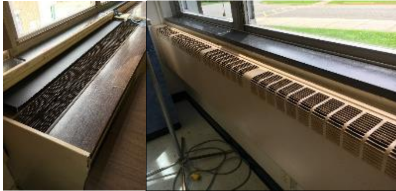
Hot Water System
