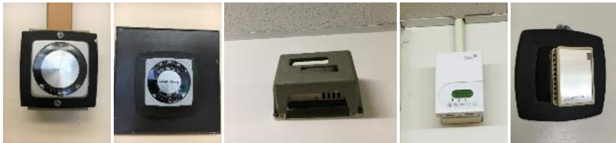
Office, Classroom and Hallway Manual Dial Thermostats (Unknown functionality, may be used solely as temperature sensors that feedback to the EMS)
