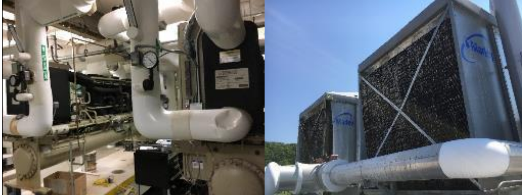
Chilled Water System
