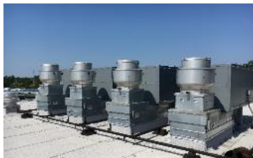
Roof Top Equipment
