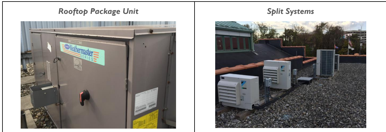
Figure 13 – Direct Expansion AC System
