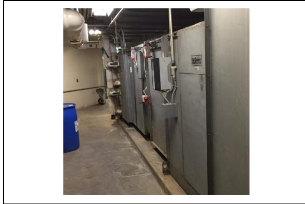
Figure 11 – Air Handling Unit
