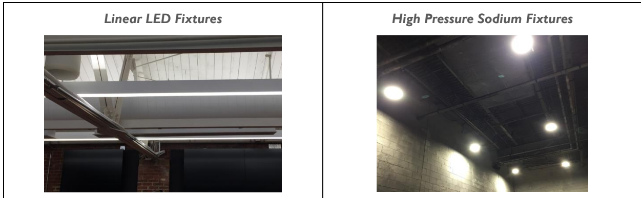
Figure 8 - Building Lighting Systems
